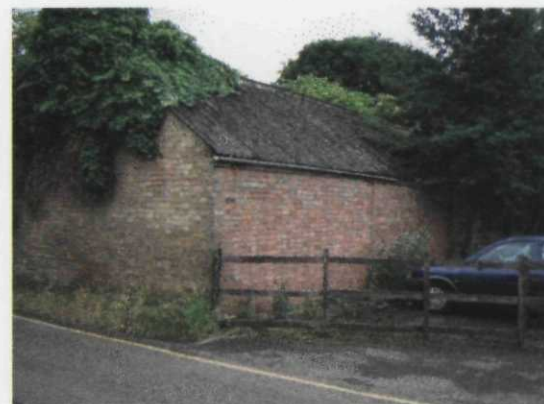
8 View across school car park
