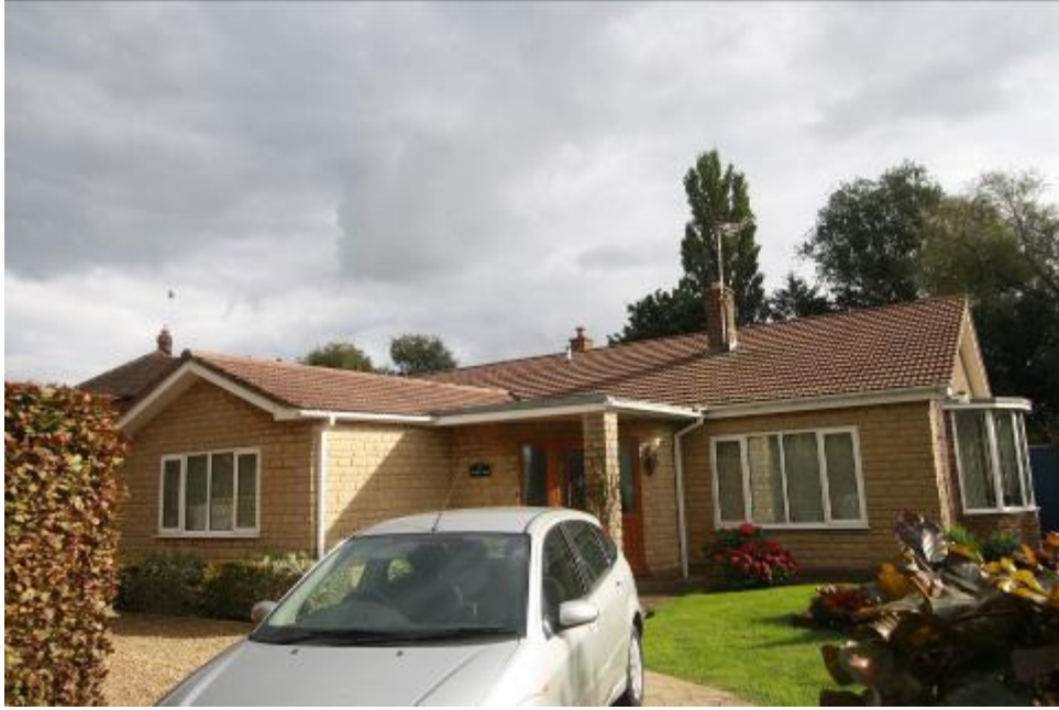
Stone Property on Low Road
