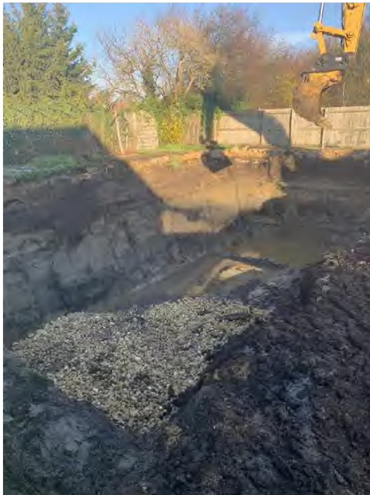
Plate 38: Placement of imported limestone aggregate in excavation base
