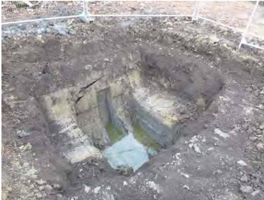
Plate 43: Completed Hotspot B (BH206) remedial excavation
