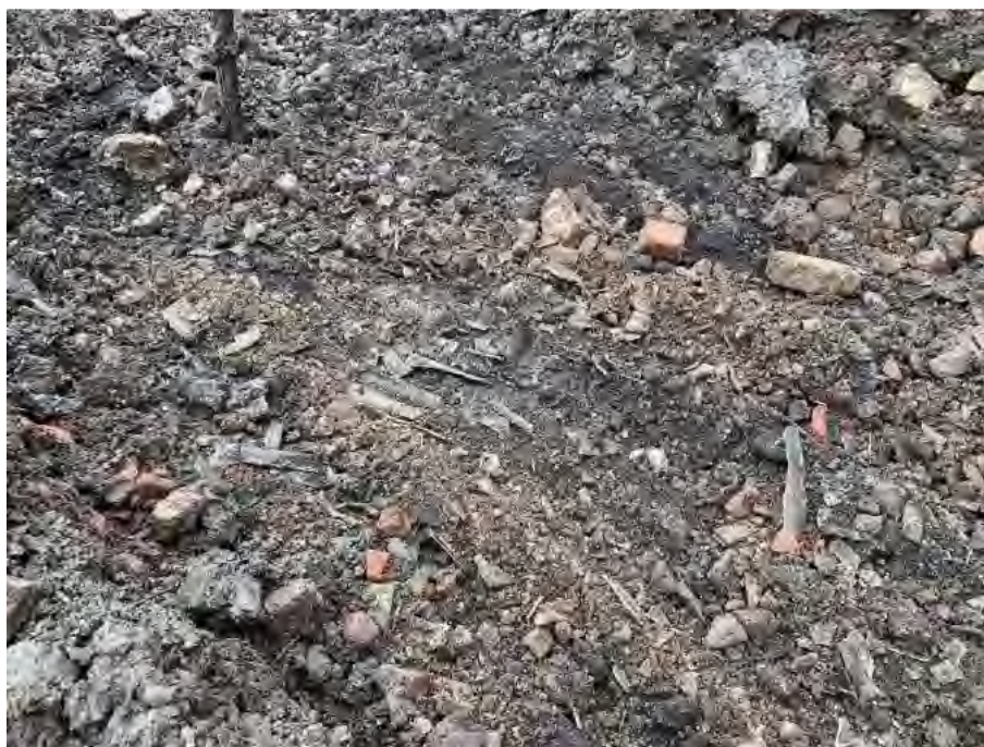
Plate 42: Asbestos cement tile fragments encountered in upper 0.5m of Hotspot B (BH206) remedial excavation – materials excavated and exported off site to
