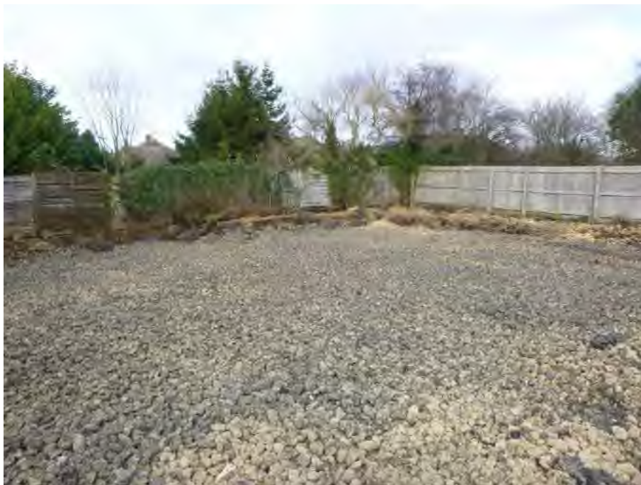
Plate 40: Imported limestone placed in 200mm layer at top of Hotspot A remedial excavation
