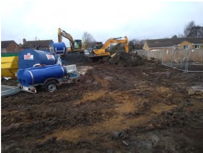
general works area
