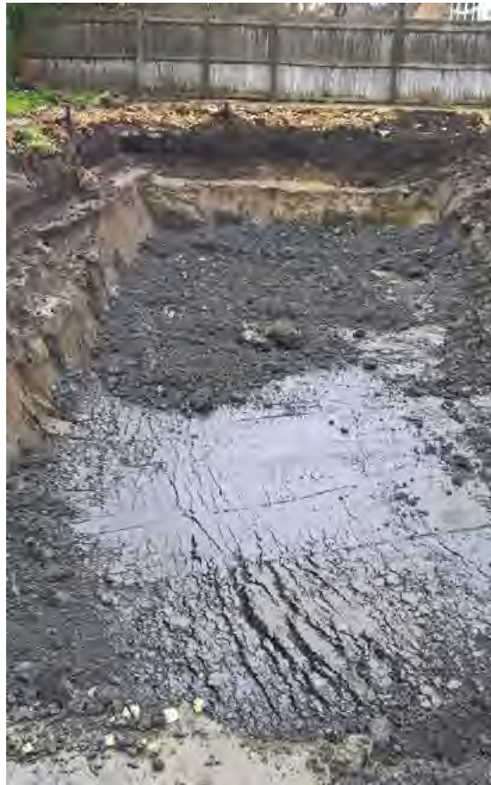
Plate 39: Placement of imported clay in Hotspot A remedial excavation
