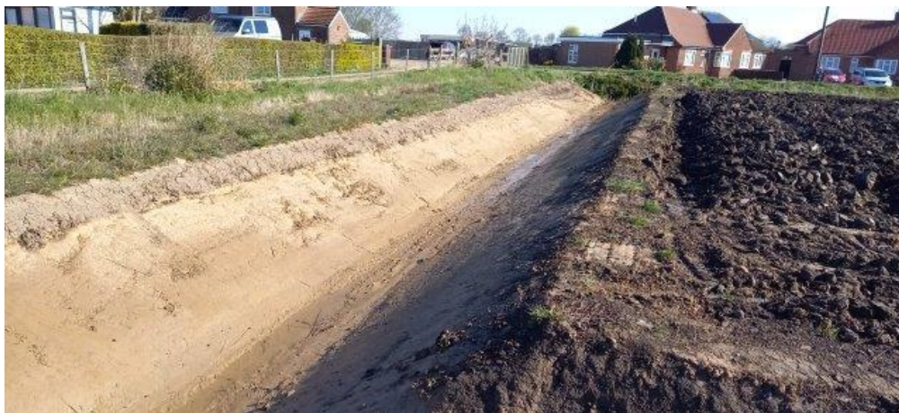
Plate 50: View of the drainage dyke at the western end of the assessment site, from the south
