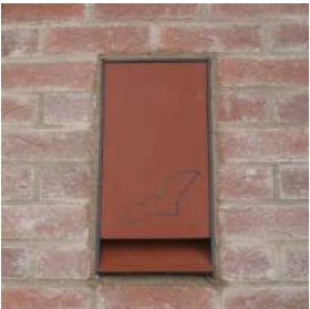
Integrated ECO Bat Boxes 1 no Cavity & 1 no Crevice
