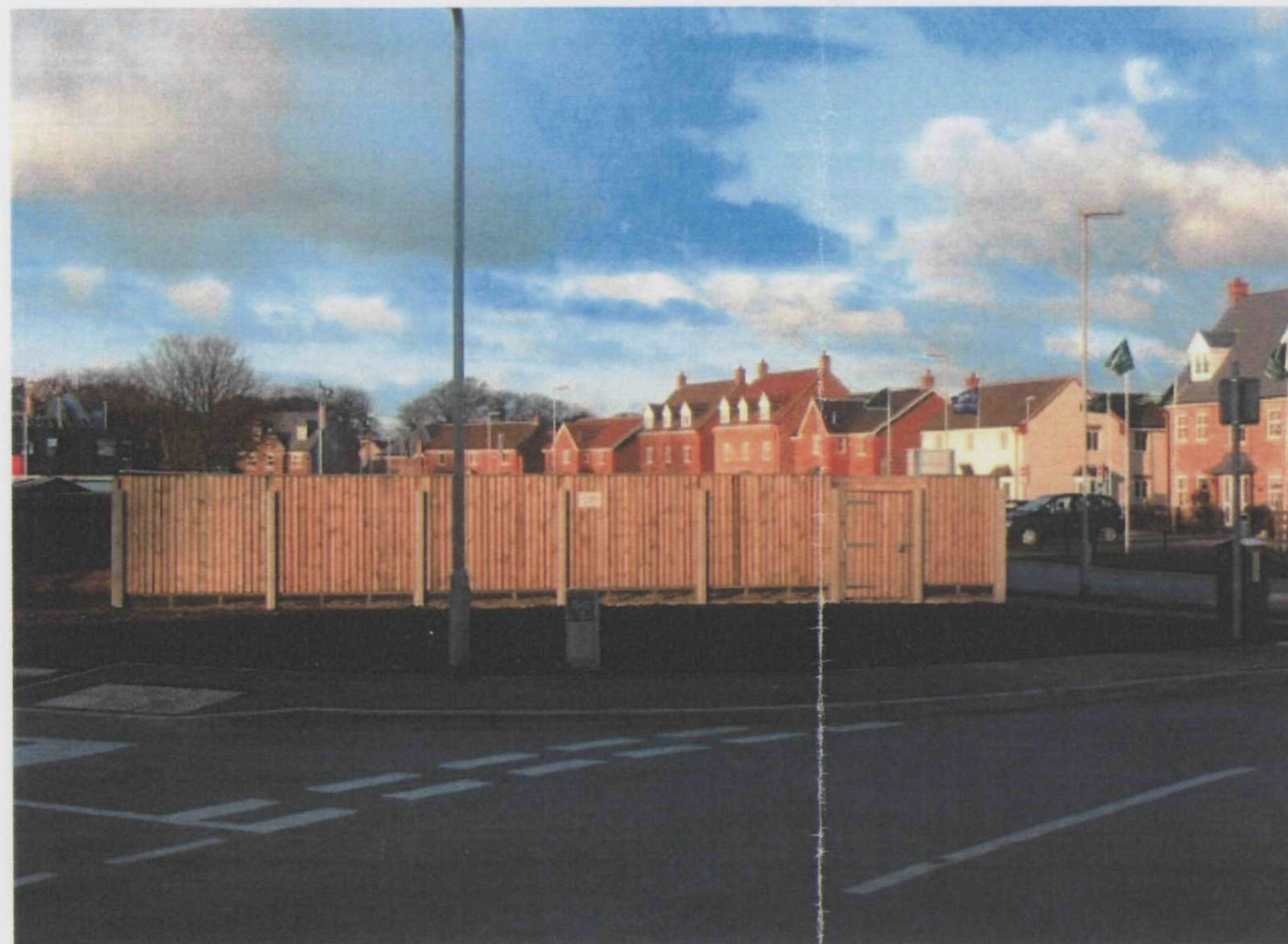
LPG Tank Compound 1 – View from South
