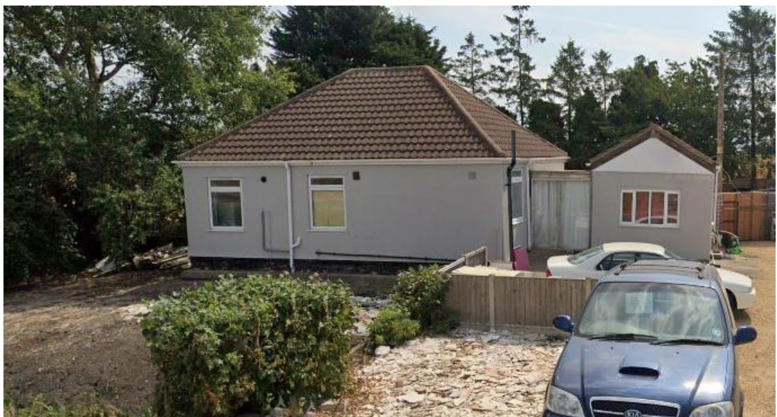
Fig 3 First property to the north east of the application site
