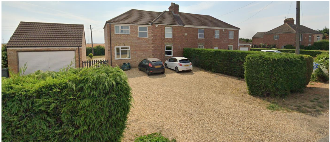
Fig 2 Properties south west of the application site
