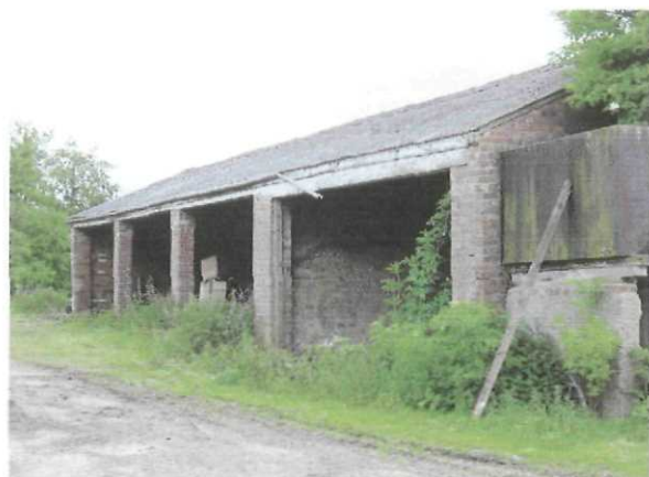
Front view of existing Agricultural building
