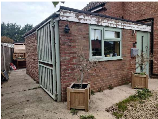
Figure 1 – Photograph of existing building.
