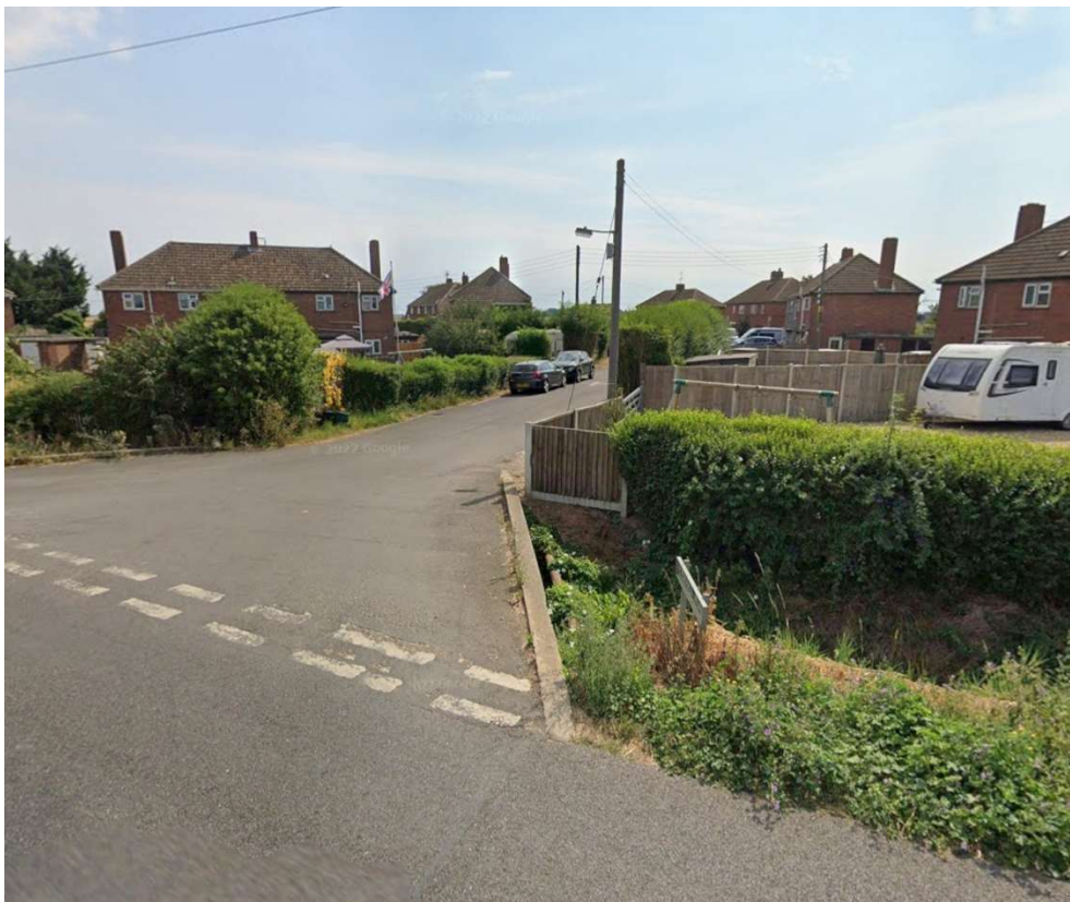
Figure 5 – Entrance to Everard Road showing no view of property from Counter Drain Drove.
