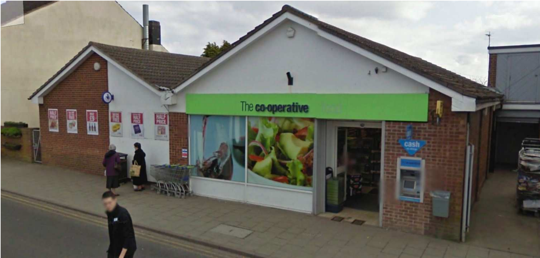
Image prior to the shop front damage (Google Street View)
