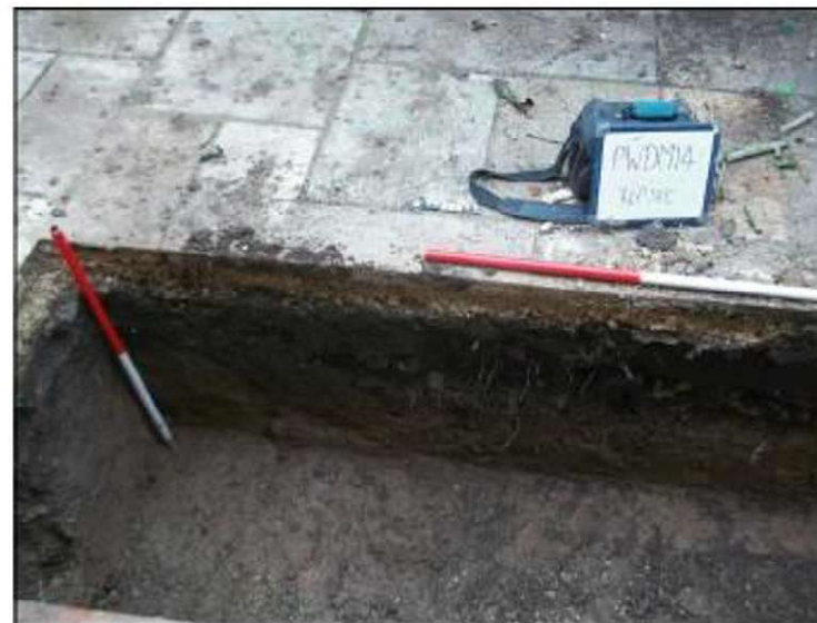
Plate. 2: Looking north-east at the northern foundation excavations
