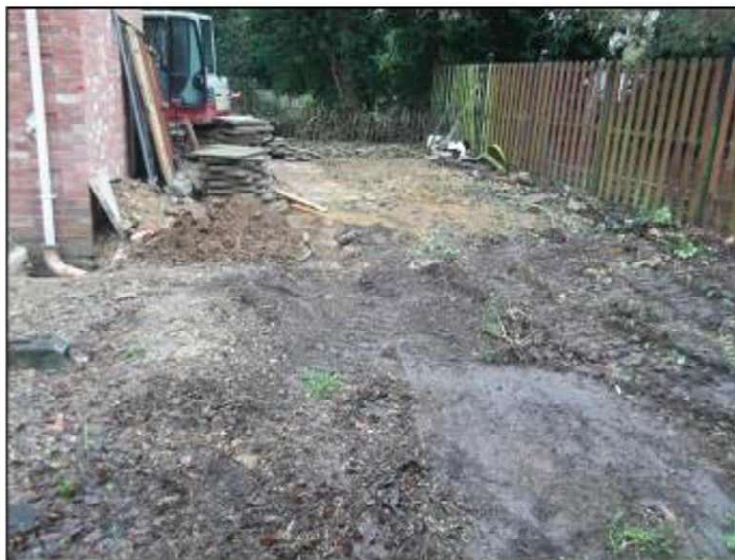
Plate. 1: Looking east pre-excavation during site clearance works
