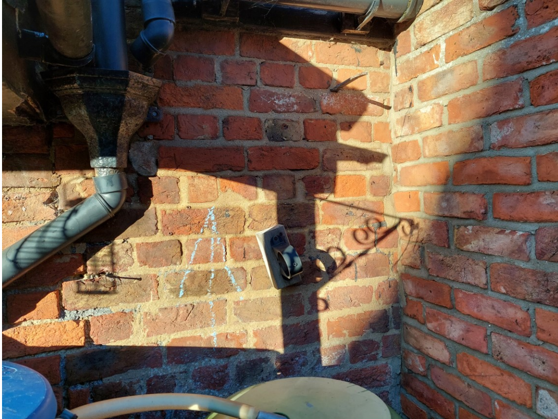
Fig. 04 – Existing outbuilding chalk height mark of original brickwork height. Adjacent addition projection / alteration.
