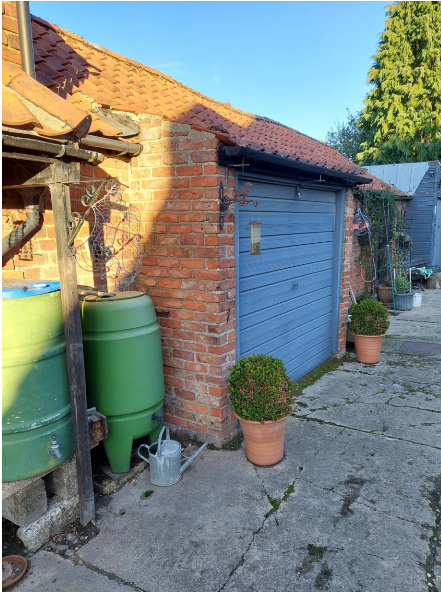
Fig. 08 – Existing single storey garage door bay projection.
