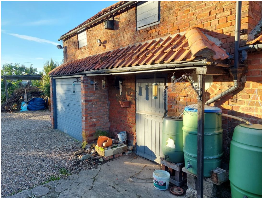
Fig. 06 – Existing brick storage building with modern addition. (Recent Photo)
