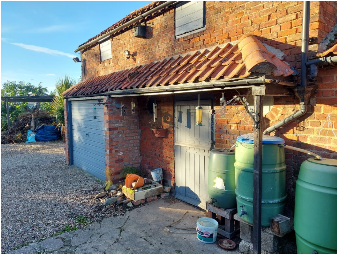
Fig. 02 – Garage and Storage Ancillary Outbuilding To Southview, Donington viewed from the south-east side.
