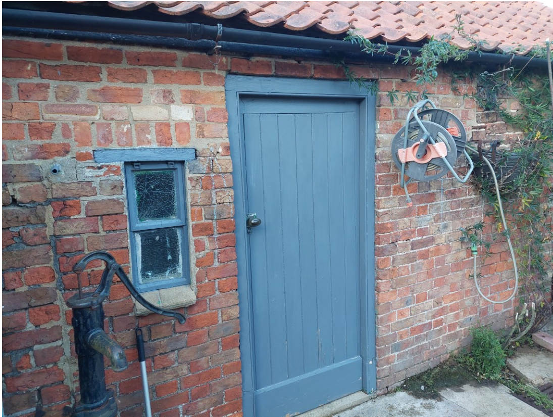
Fig. 05 – Existing brick outbuilding.
