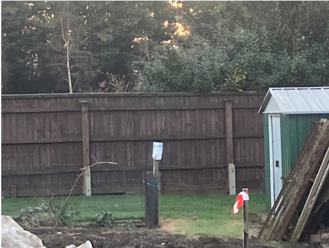
Fig. 09 – Existing east boundary to POS with high Close Boarded Fence,
