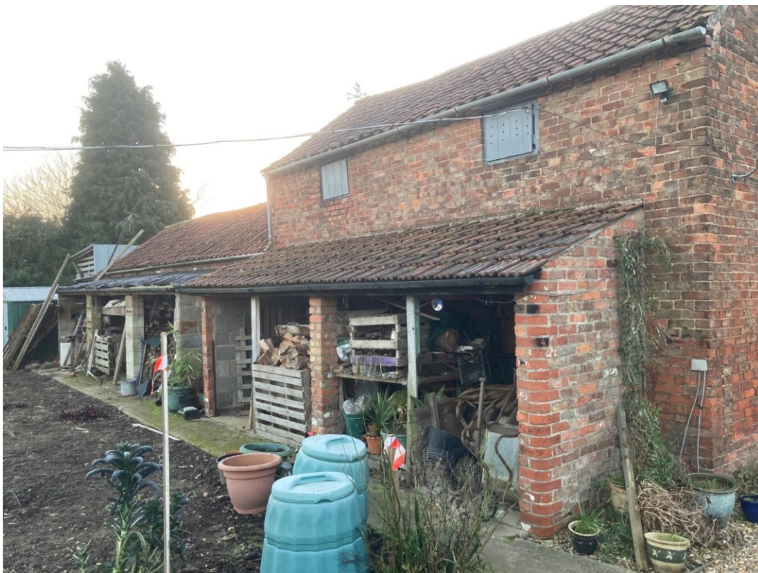
Fig. 03 – Garage and Storage Ancillary Outbuilding To Southview, Donington viewed from the North-West side.
