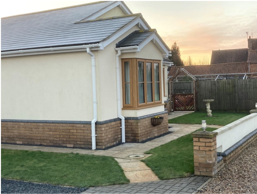
Fig. 12 – 10 Goxhill Avenue, Cream Render, Buff brick plinth and modern slates. View from the Northwest.
