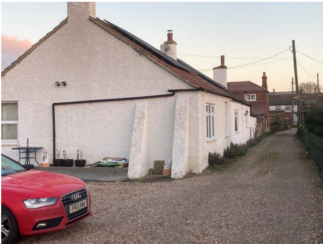
Fig. 11 – 11 Goxhill Avenue, White Painted Render Bungalow. View from the Southeast.
