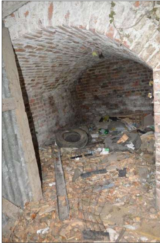
Plate 76 (shot 127): Vaulted storage space in C0.7. Looking east-northeast
