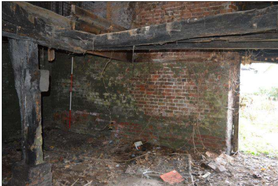
Plate 74 (shot 122): General view toward the west, showing reclaimed timbers. Looking west-southwest, 2m scale
