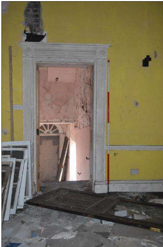
Plate 38 (shot 162): Doorway into the Assembly Room. Looking west-northwest, 2m scale
