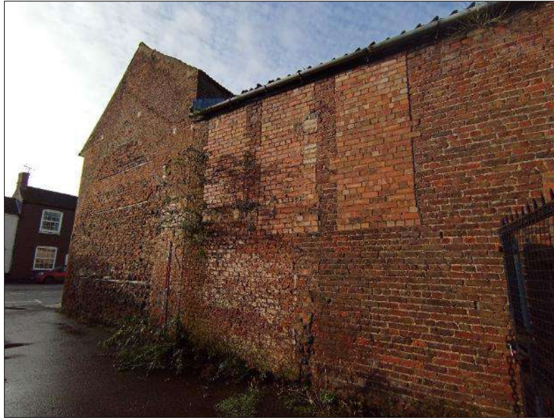
Plate 48 (shot 170): Straight joint between Structures B and C and blocked up, later, tall windows. Looking south-southwest, 2m scale
