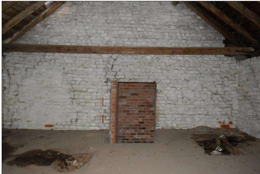
Plate 82 (shot 277): Partition and loft entrance between C.1.1, notice blocked opening above the staircase.
