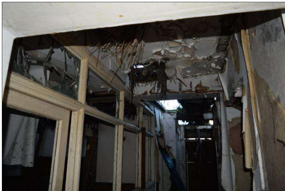
Plate 87 (shot 200): Ground floor corridor and function room, showing reeded and plastered ceiling. Looking northwest
