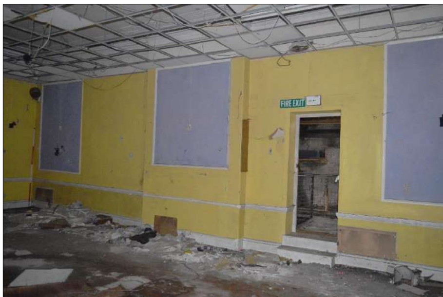
Plate 42 (shot 157): North wall showing chimney breast with blocked fireplace and a doorway to Structure C. Looking north-northwest, 2m scale
