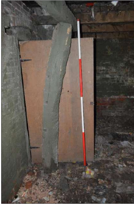
Plate 75 (shot 121): Reclaimed curved timber supporting beam above. Looking south-southwest, 2m scale
