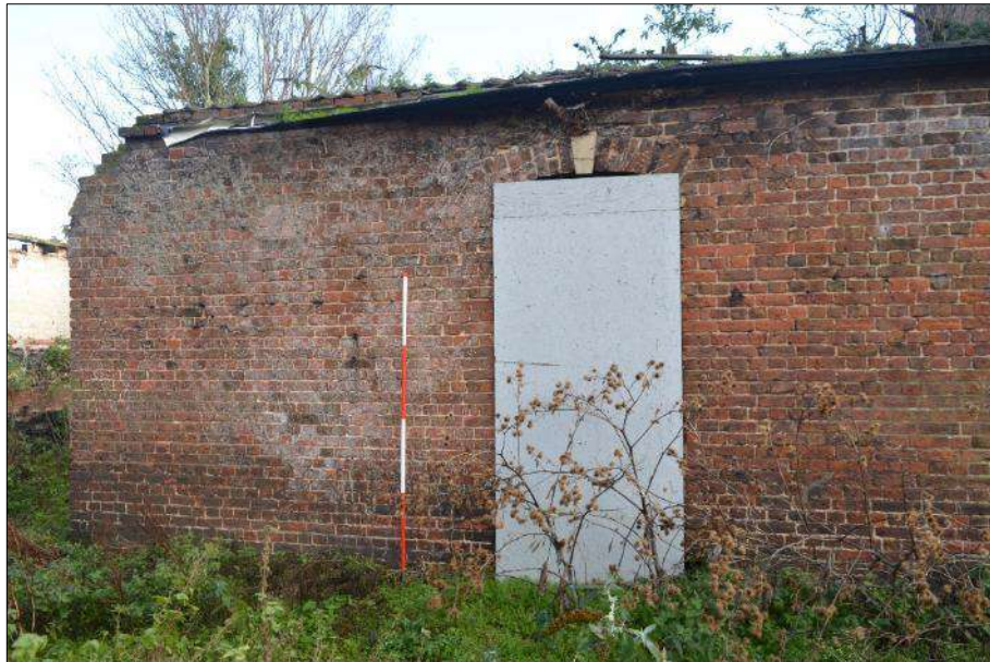
Plate 56 (shot 42): West elevation with boarded up doorway of C0.1. Looking east-southeast, 2m scale
