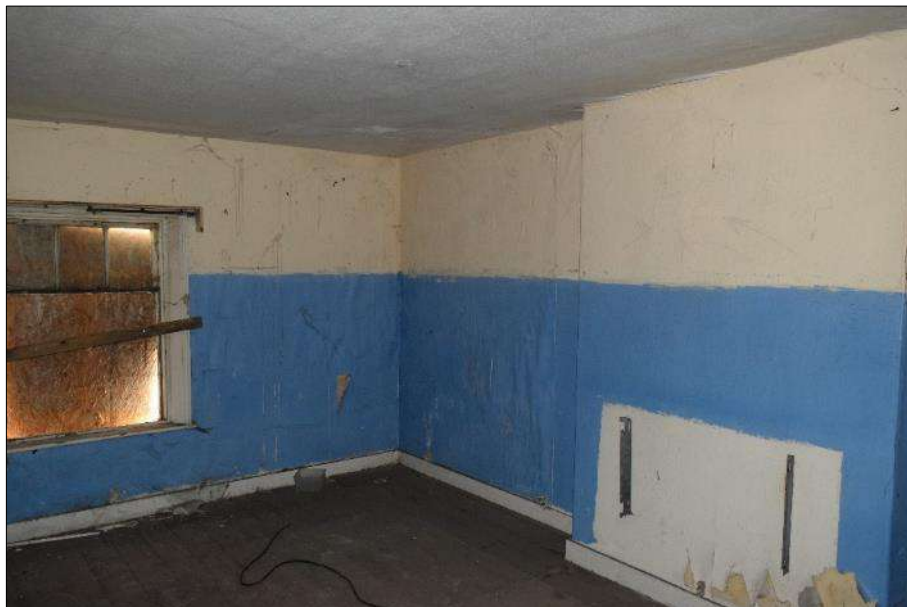
Plate 30 (shot 261) Room A2.1 showing blocked fireplace. Looking southwest
