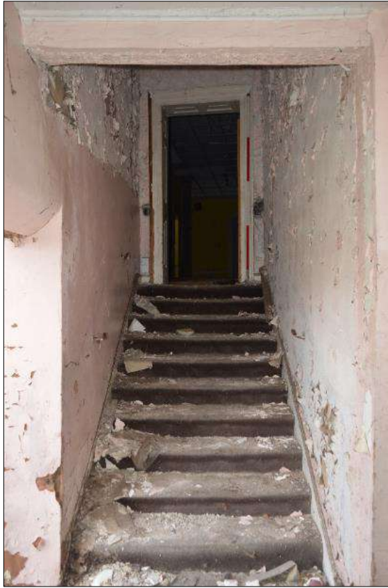
Plate 37 (shot 144): General view of the Assembly Room staircase. Looking east, 2m scale
