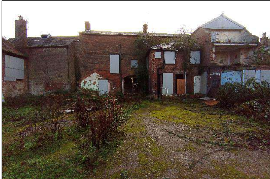
Plate 7 (shot 175): General view of the rear of the hotel also showing Structures B, C and D. Looking south, 2m scale
