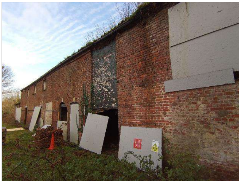
Plate 53 (shot 174): Oblique view of west elevation. Looking north-northeast, 2m scale
