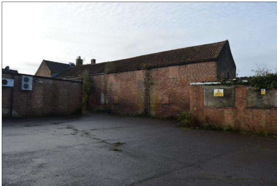
Plate 49 (shot 172): East elevation of Structure C. Looking northeast, 2m scale
