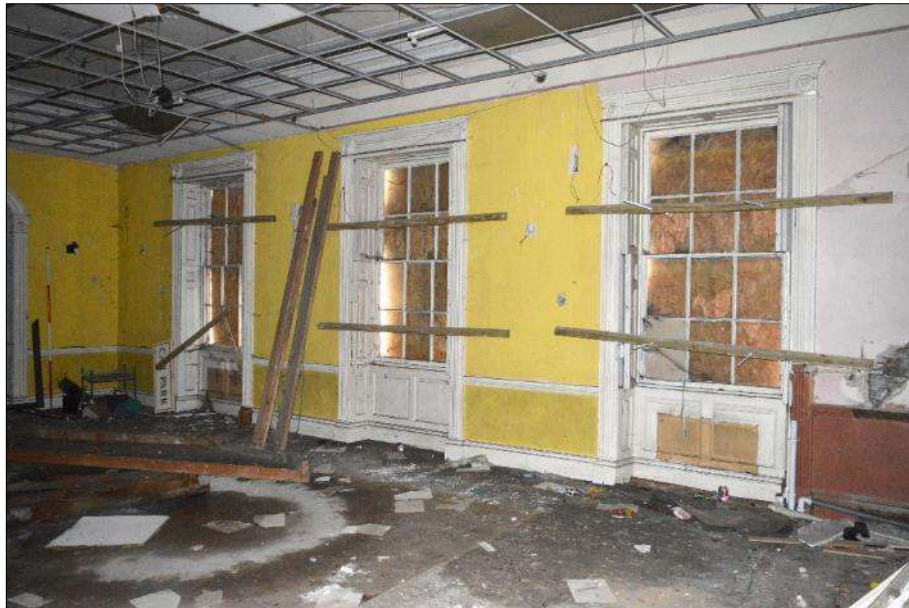
Plate 39 (shot 155): Georgian windows in the Assembly Room. Looking southeast, 2m scale
