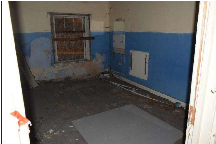
Plate 31 (shot 258): Bedroom A2.2. Looking southwest
