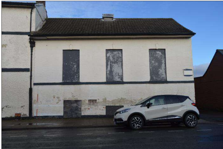
Plate 33 (shot 23): The Assembly Room fronting the High Street. Looking north-northeast, 2m scale
