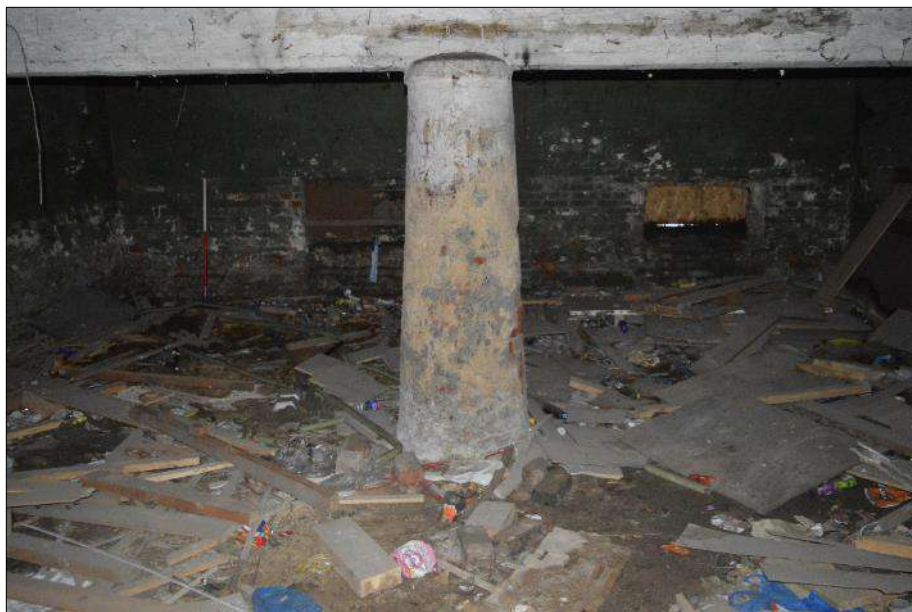
Plate 46 (shot 128): View of the ground floor room to the south. Looking north-northeast, 1m scale
