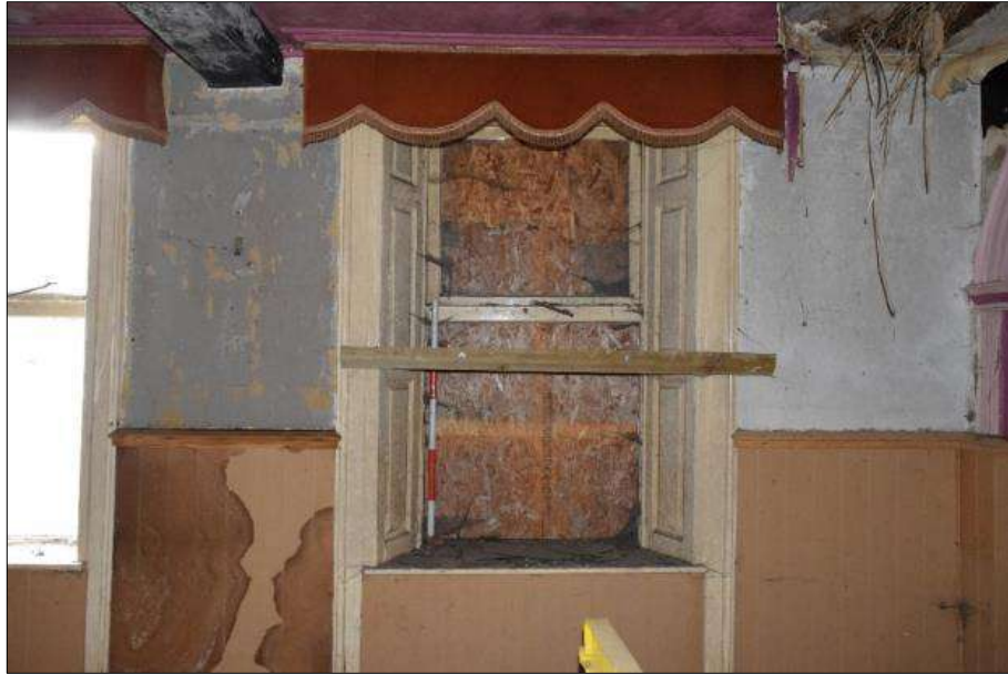
Plate 15 (shot 191): Close up of window with shutters. Hole in the ceiling displays plaster over reeds. Looking south, 1m and 0.5m scale
