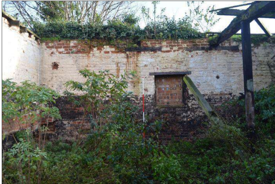
Plate 60 (shot 35): Interior view of C0.1, showing blocked window with segmental arch. Looking east-southeast, 2m scale
