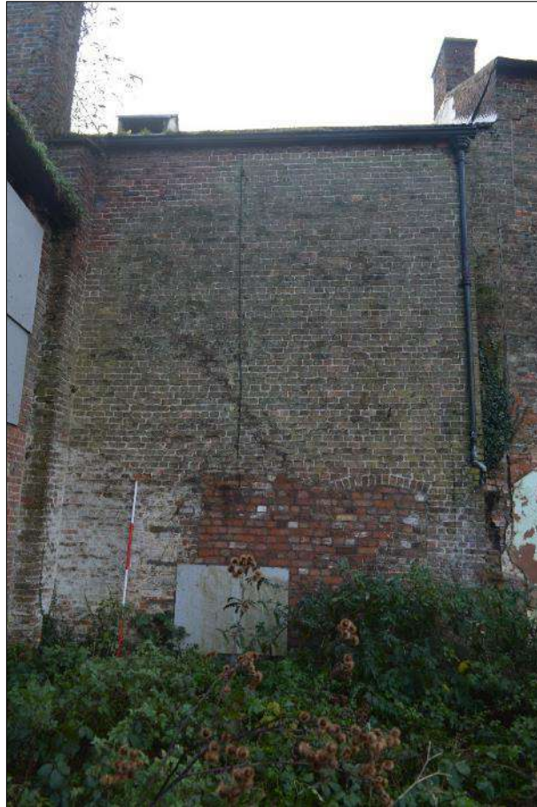
Plate 36 (shot 61): North elevation of Structure B, showing blocked doorway. Looking south-southwest, 2m scale
