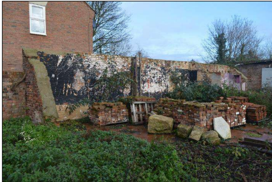
Plate 88 (shot 168): General view of the remains of Structure E. Looking northeast, 2m scale
