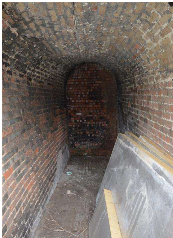
Plate 70 (shot 117): Blocked off archway C0.6. Looking east-southeast
