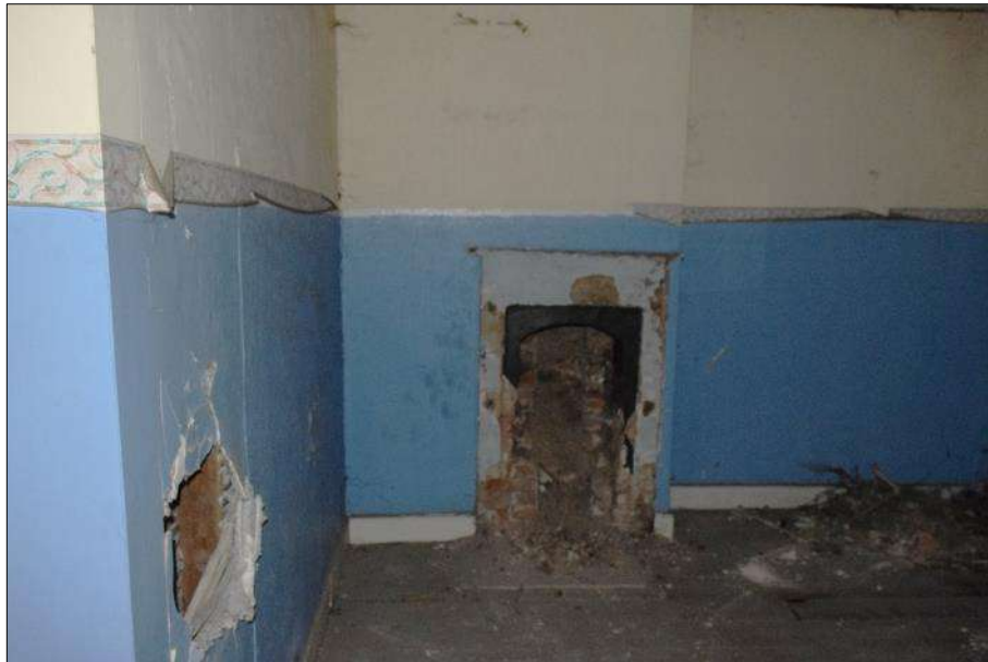
Plate 27 (shot 230): Fireplace in room A1.5 on the east wall. Looking east
