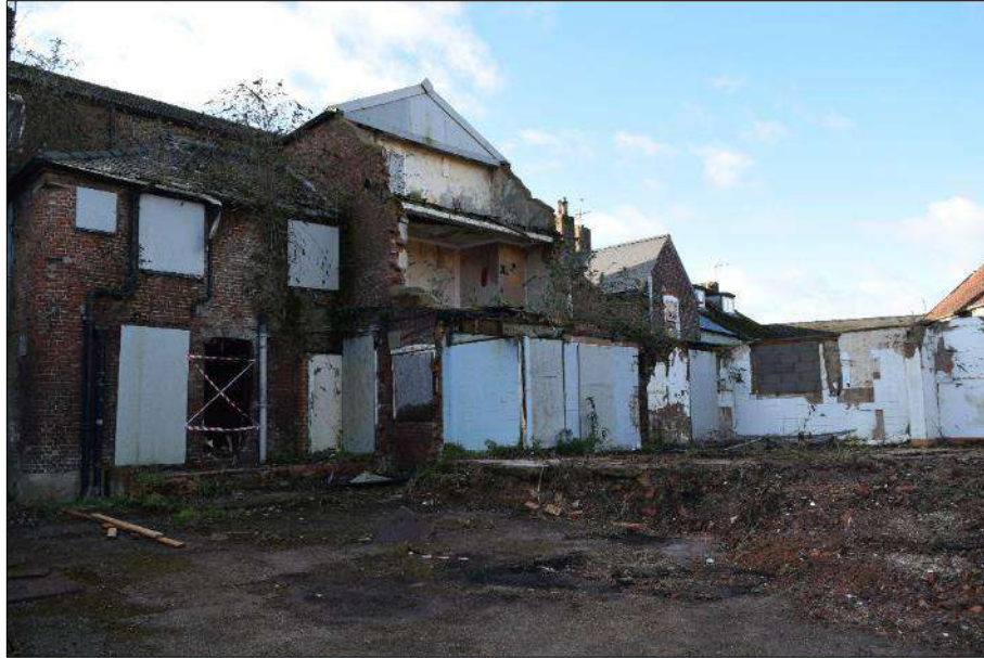
Plate 10 (shot 207): General view of extensions on north elevation. Looking southwest
