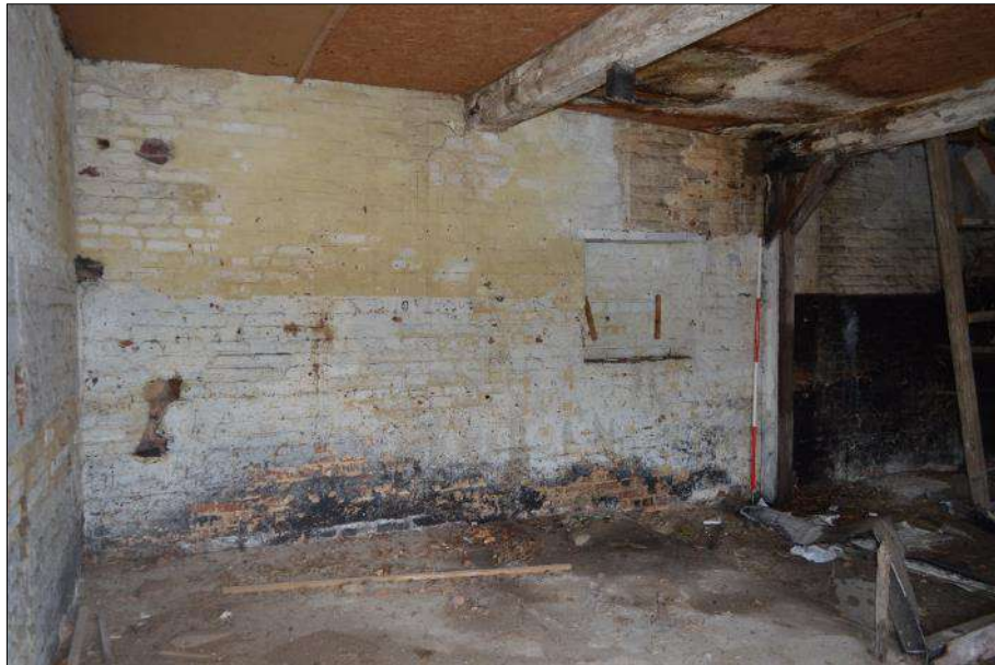
Plate 67 (shot 110): View across the north area in C0.5, showing modern floor, removed timber post and blocked window. Looking southeast, 2m scale
