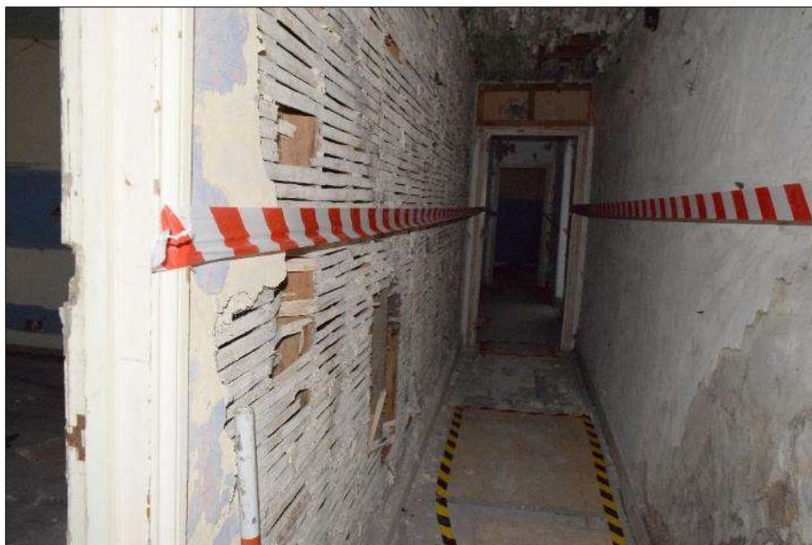
Plate 28 (shot 251): View along the second floor corridor. Looking west
