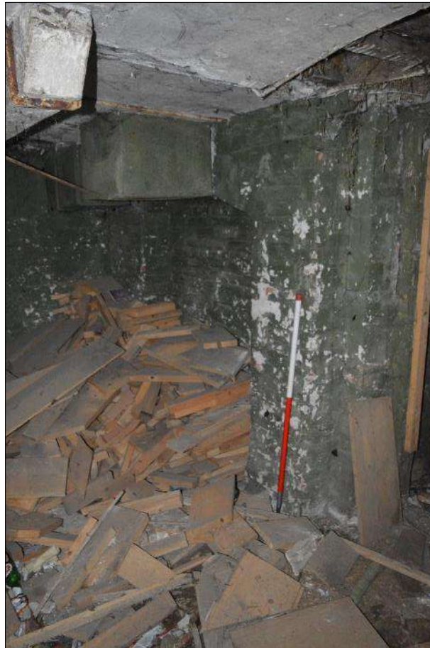
Plate 47 (shot 134): Segmental arched niche and removed fireplace. Looking north-northwest, 1m scale
