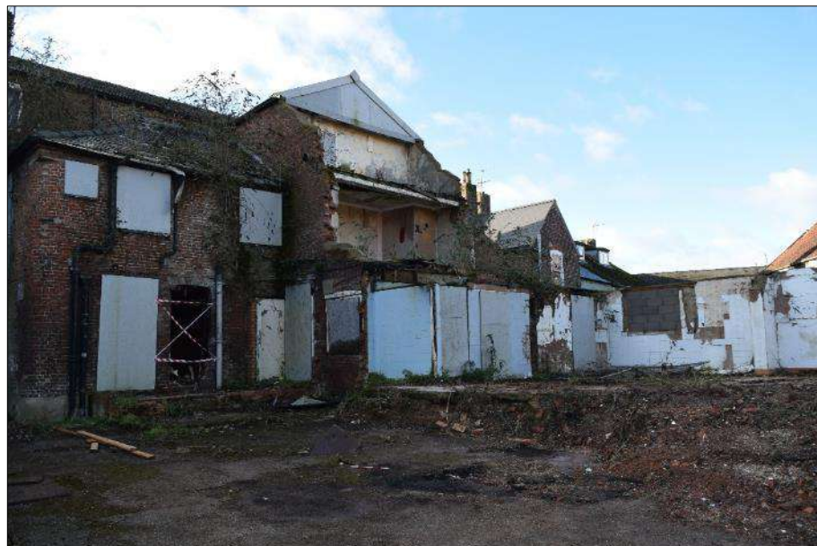
Plate 85 (shot 207): General view of partially demolished north wing D. Looking southwest
