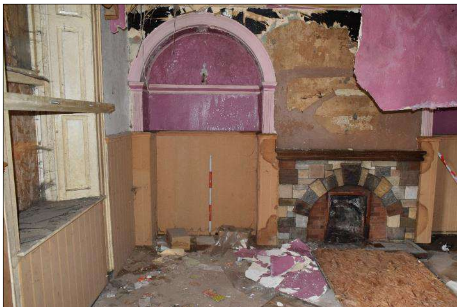
Plate 14 (shot 194): General view of western bar area showing alcove and modern fireplace. Looking west, 1m scale
