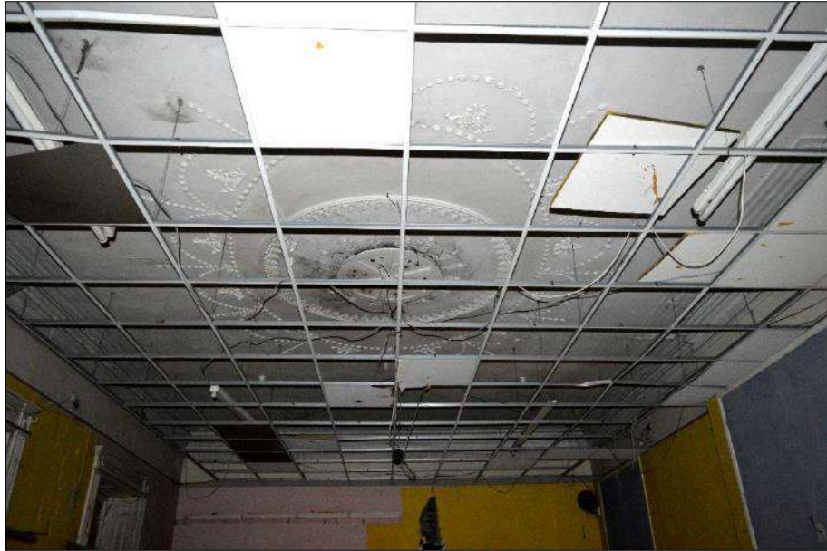
Plate 43 (shot 160): Plastered ceiling with floral motif and plastered cornice. Looking west-northwest
