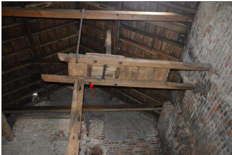
Plate 79 (shot 139): Platform above north mezzanine, arrow points to circular cut hole in a square platform fixed in position by square nots and bolts/tails. Looking north-northeast
