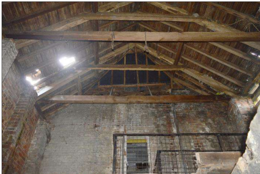
Plate 81 (shot 137): View towards the south mezzanine showing the roof structure. Looking south-southwest
