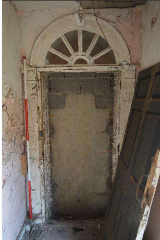
Plate 16 (shot 142): Georgian architrave and main former entrance to the assembly room. Looking west-northwest, 2m scale
