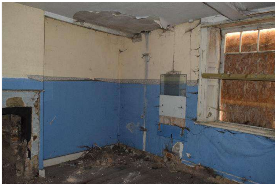
Plate 26 (shot 231): General view of room A1.5. Looking southeast
