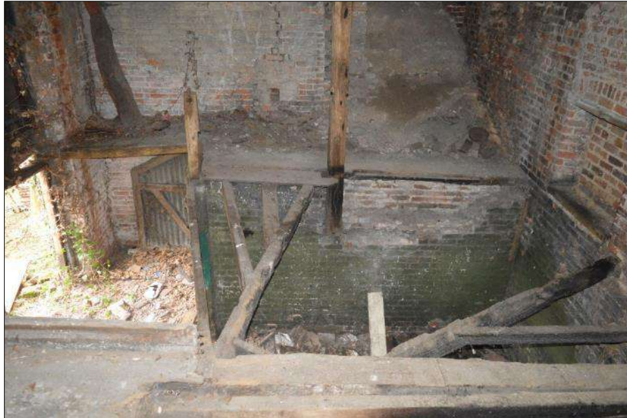
Plate 80 (shot 153): Close up of mezzanine and branching floor structure. Looking north-northeast
