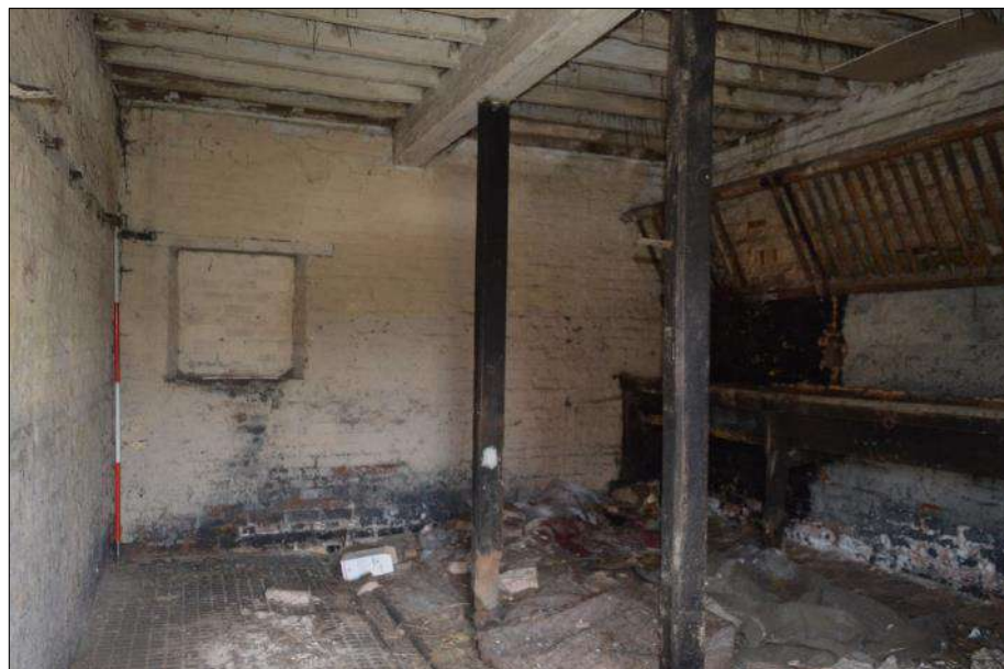
Plate 66 (shot 98): General view of C0.4 towards the east wall with blocked window, also showing retained original features. Looking east-southeast, 2m scale
