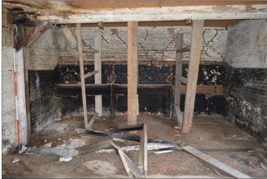
Plate 69 (shot 111): View towards the south end of C0.5, showing herringbone brick floor, amended trough, modern supporting timber frames and hewn original main beam and diagonal brace.
