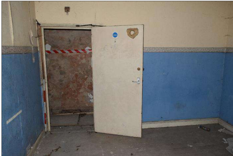
Plate 25 (shot 235): General view towards the corridor from room A1.4. Looking north, 1m scale
