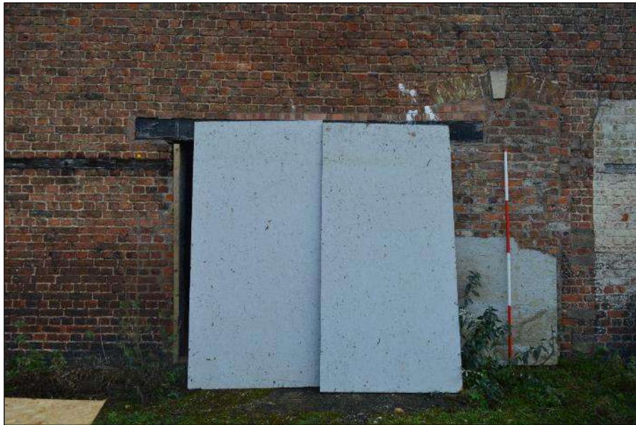
Plate 58 (shot 52): Bricked up doorway replaced with boarded up cart opening. Looking east-southeast, 2m scale
