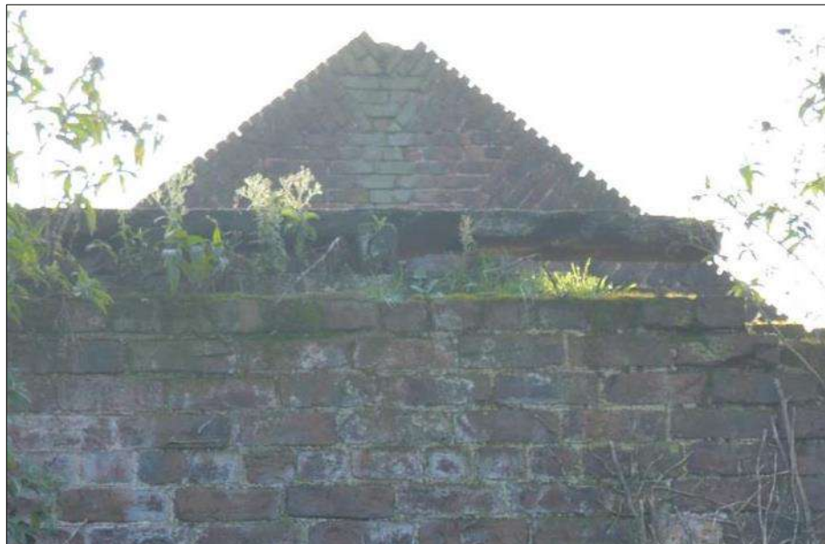
Plate 51 (shot 34): Close-up of tumbled brickwork in the background on the north gable. Looking south-southwest
