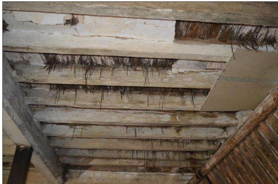
Plate 64 (shot 102): Close up of plastered ceiling in C0.4. Looking north
