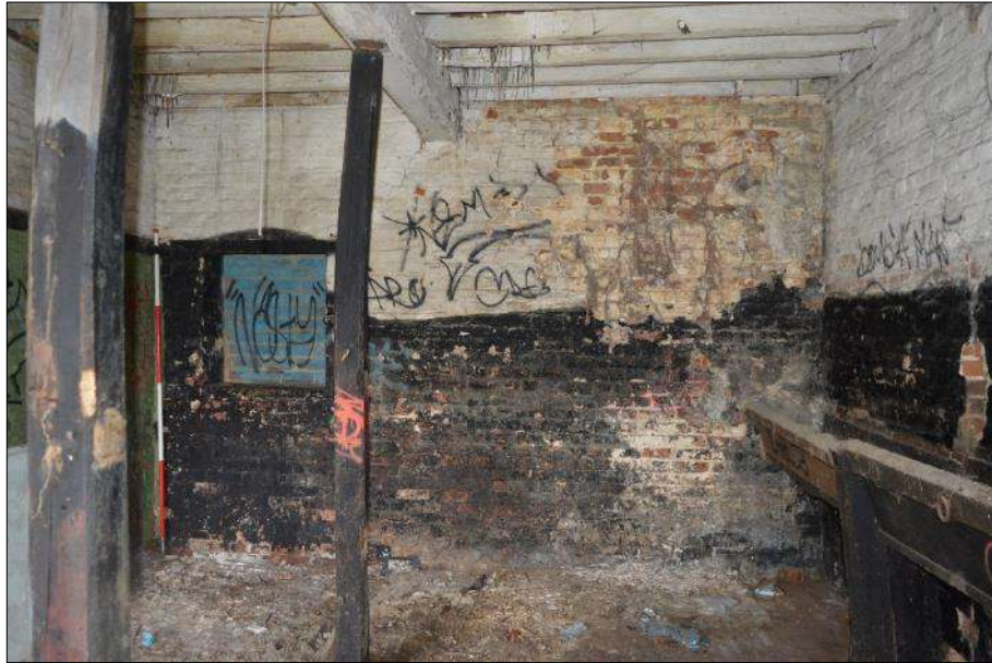
Plate 62 (shot 85): General view of stable C0.3. Looking east-southeast, 2m scale
