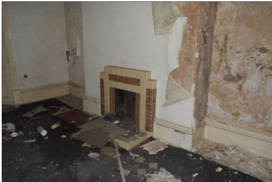
Plate 22 (shot 215): Fireplace in bedroom A1.1. Looking west-southwest
