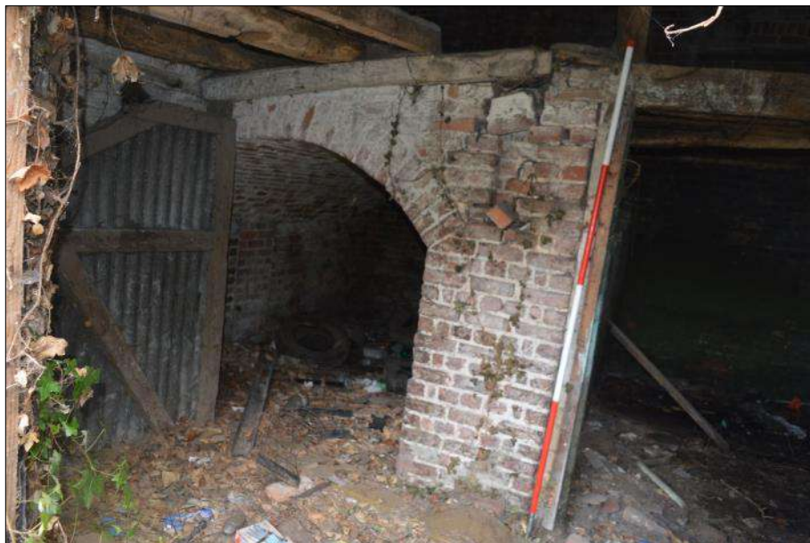
Plate 77 (shot 125): General view towards the vaulted storage room in C0.7. Looking east-northeast, 2m scale
