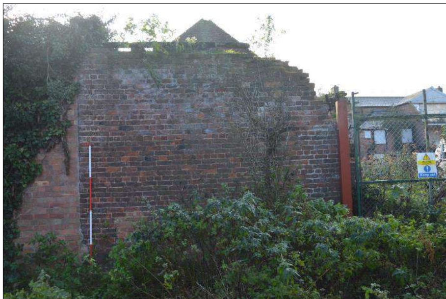
Plate 55 (shot 34): North elevation of C0.1 showing modern building to the left. Looking south-southwest, 2m scale.
