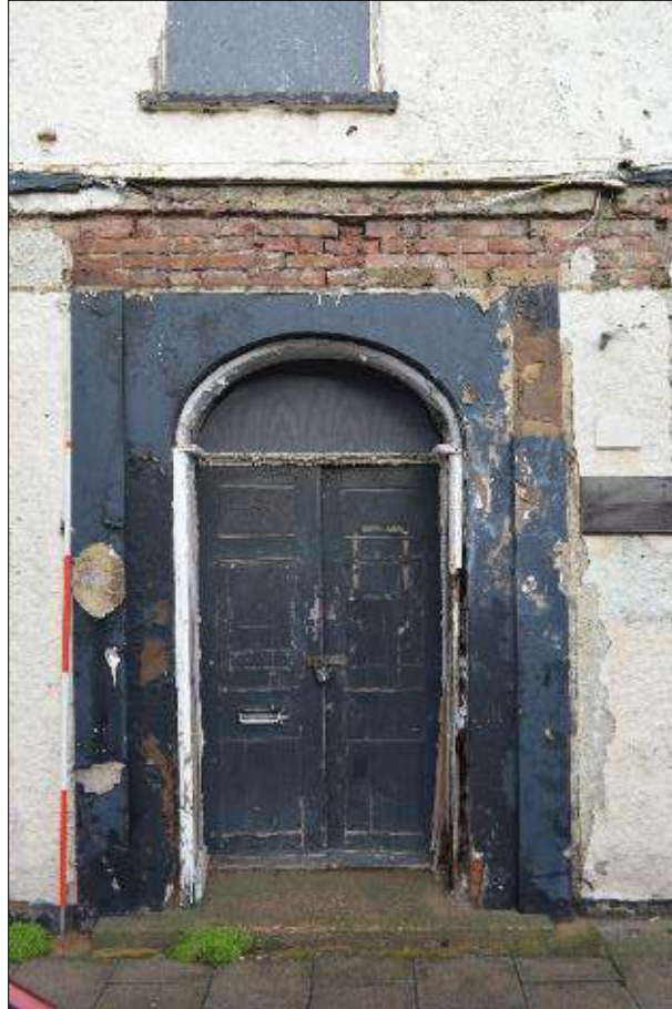
Plate 4 (shot 17): Main entrance. Looking north, 2m scale
