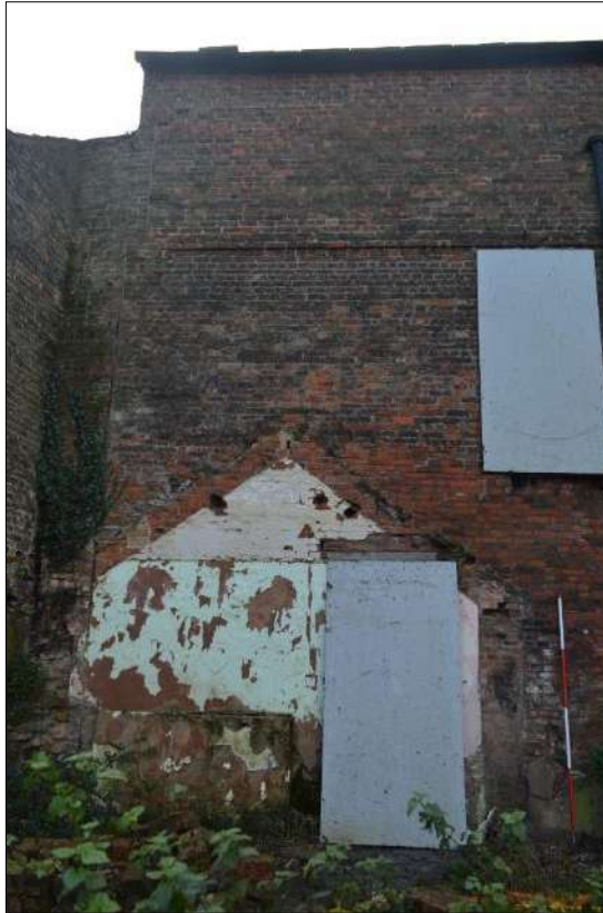
Plate 8 (shot 64): Scarring of removed structure on the north elevation, also showing ragged joint on second floor. Looking south, 2m scale
