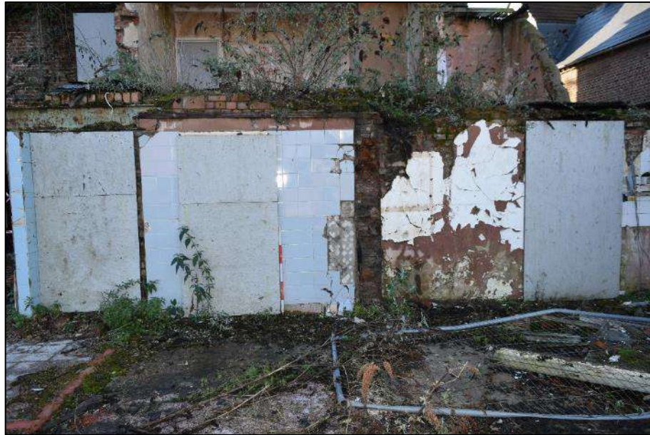
Plate 86 (shot 203): General view of demolished areas of D. Looking south, 1m scale
