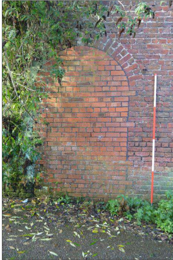
Plate 50 (shot 32): Blocked archway on the east elevation. Looking west, 2m scale
