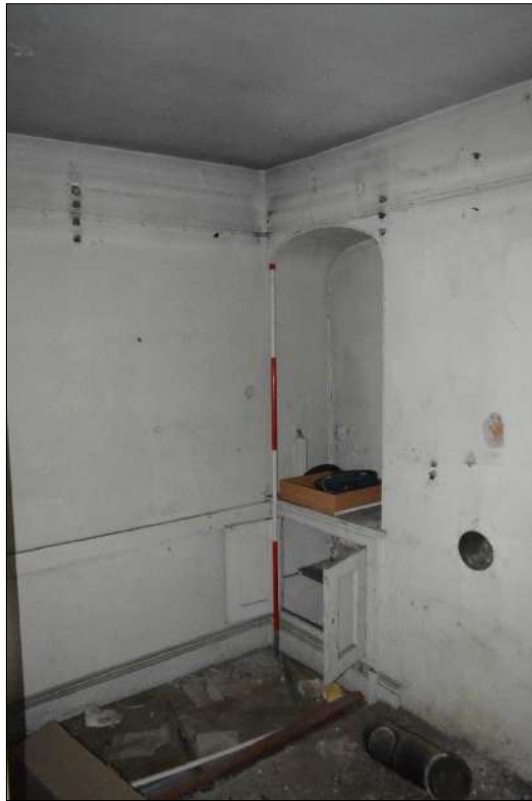
Plate 17 (shot 149): Niche with built-in cupboard and flue hole in the eastern wall. Looking northeast, scale 2m
