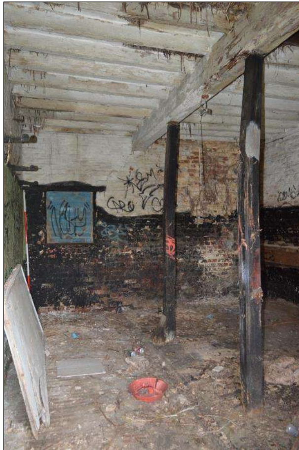
Plate 63 (shot 83): View of C0.3 showing harness pegs on the north wall, and brick floor. Looking east, 2m scale
