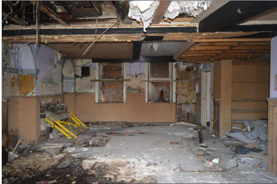
Plate 11 (shot 164): General view of eastern bar/reception area. Looking south
