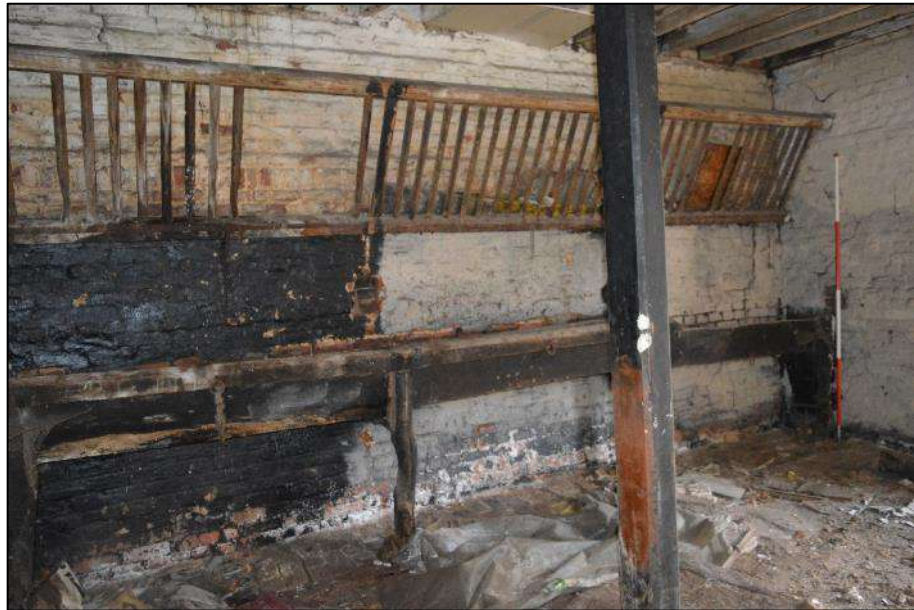
Plate 65 (shot 104): Close up of wooden trough and hayrack in C0.4. Looking west-southwest, 2m scale
