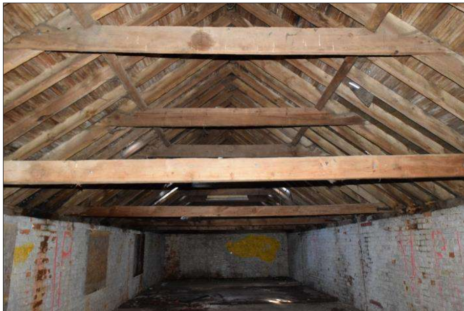
Plate 83 (shot 275): General view along loft, C1.2, showing timber roof structure. Looking north-northeast
