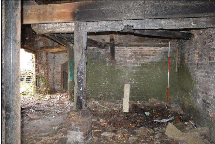
Plate 73 (shot 123): Heat affected timbers of C0.7. Looking north, 2m scale
