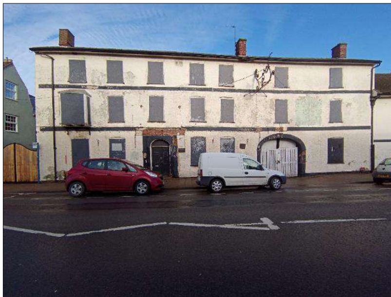
Plate 1 (shot 171): General view of the hotel from the High Street. Looking north
