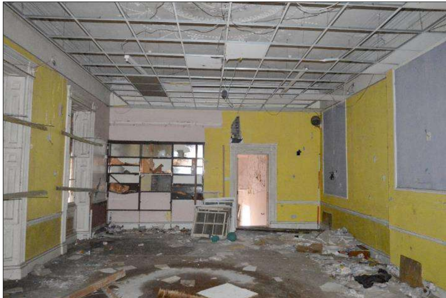
Plate 41 (shot 156): General view of the Assembly Room to the west. Looking west-northwest, 2m scale
