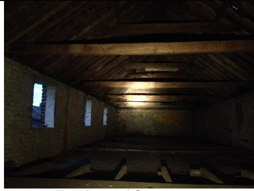
Top floor of Structure 5
