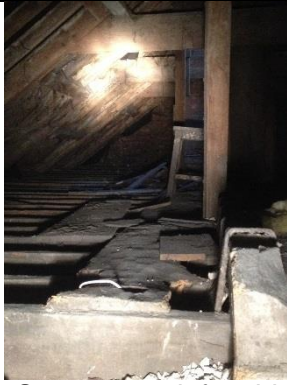
Structure 1- loft void
