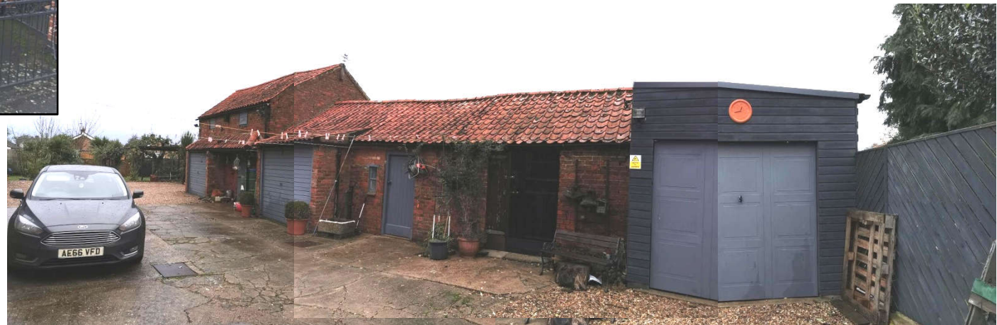
Older out-building to the north of the house. (to be demolished) – looking northwest
