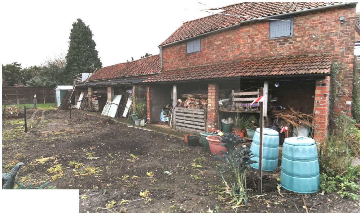
View of smaller development site to the north behind the out-building (to be demolished) – looking southeast
