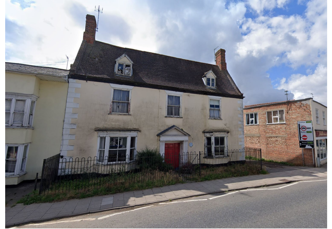
Image 8 Showing no.1 High Street—Listed Building.
