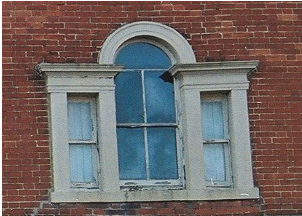
Fig 2.5 – Bricks on the front façade.
