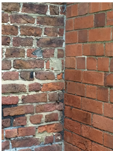
Fig 2.6 Junction between the rear façade and Victorian side annex.
