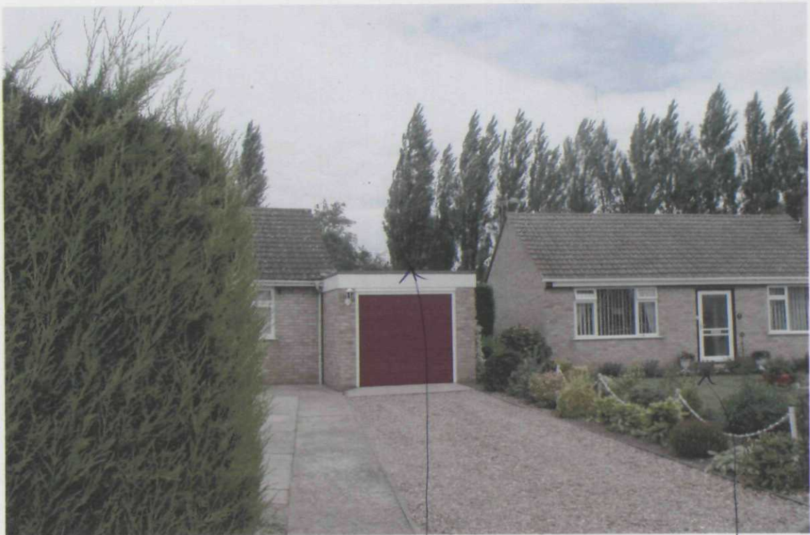
Roof to go here
