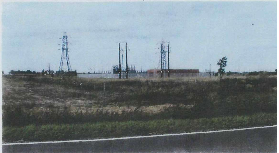
Power distribution infrastructure south of Holbeach
