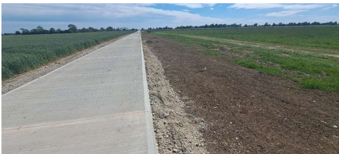
Photograph 6: Access to the application site from Fen Lane facing south at approximate OSGR TF 19077 35794
