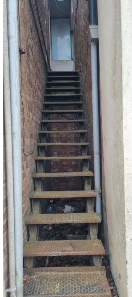
External stairway (to be fire escape).
