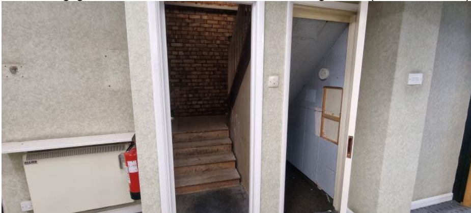
An existing ground floor storeroom and the existing stairs (to be removed).
