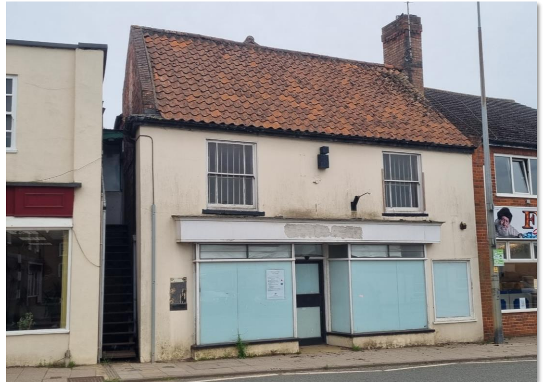
Fig 4: Photo of the application site in its current condition (vacant since 2018).
