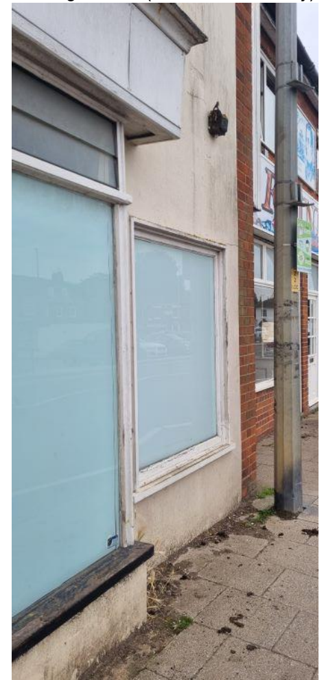
Existing window (to become doorway).
