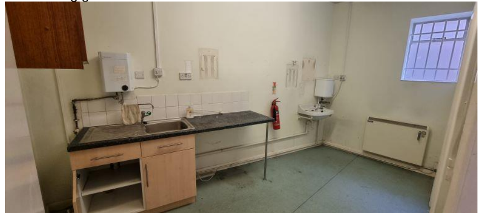
The existing ground floor kitchen is to be refitted and modernised.
