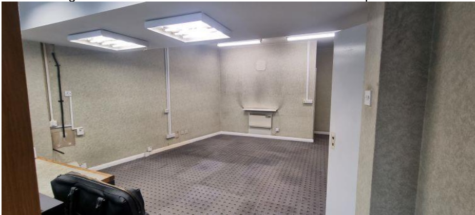
Part of the ground floor – to become multi-functional office space.
