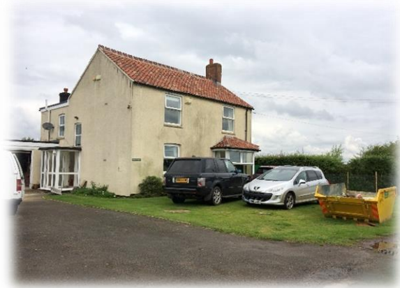
Fig.6: Photo of front elevation of Eastview showing existing grassed area to the east which is used for parking.
