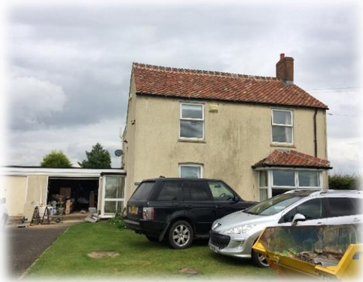
Fig.5: Photo of front elevation of Eastview showing flat roof garage and porch appended to its southern elevation
