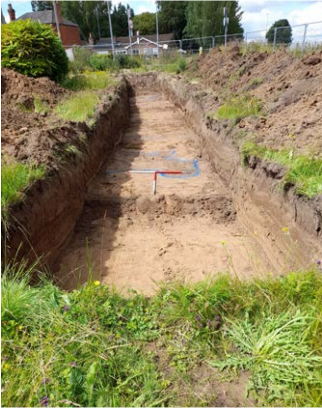
Photograph of Trench 1 from east
