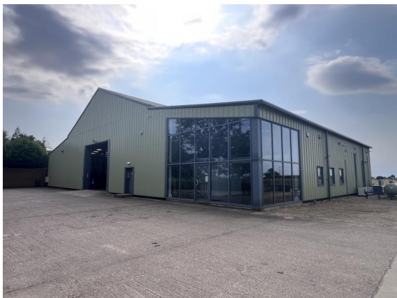
Fig. 09 – Harvey's Barn following the 2012 works.
