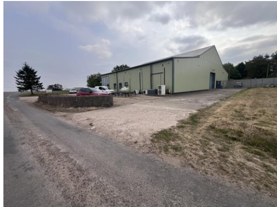
Fig. 04 – North boundary –open to Day's Lane.
