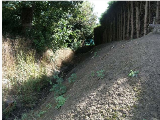
Figure 4- Two Surface water drainage ditches were identified at the eastern side of the A52 road
