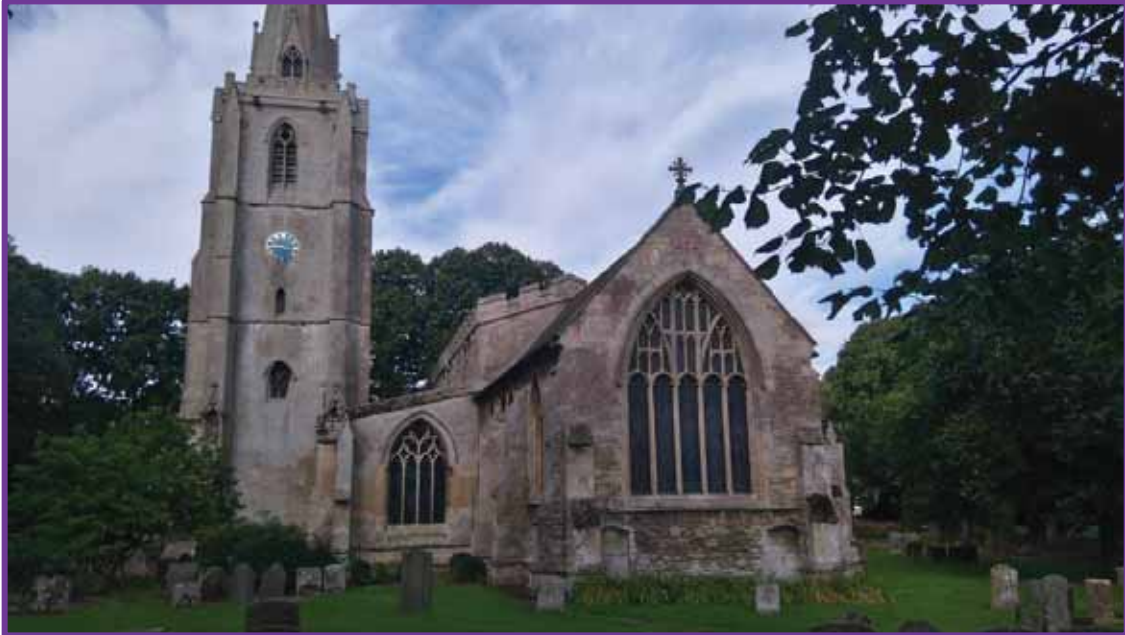
Plate 3. Church of St Mary and The Holy Rood, looking west
