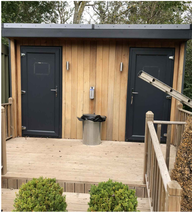
AS BUILT PHOTOGRAPHS
