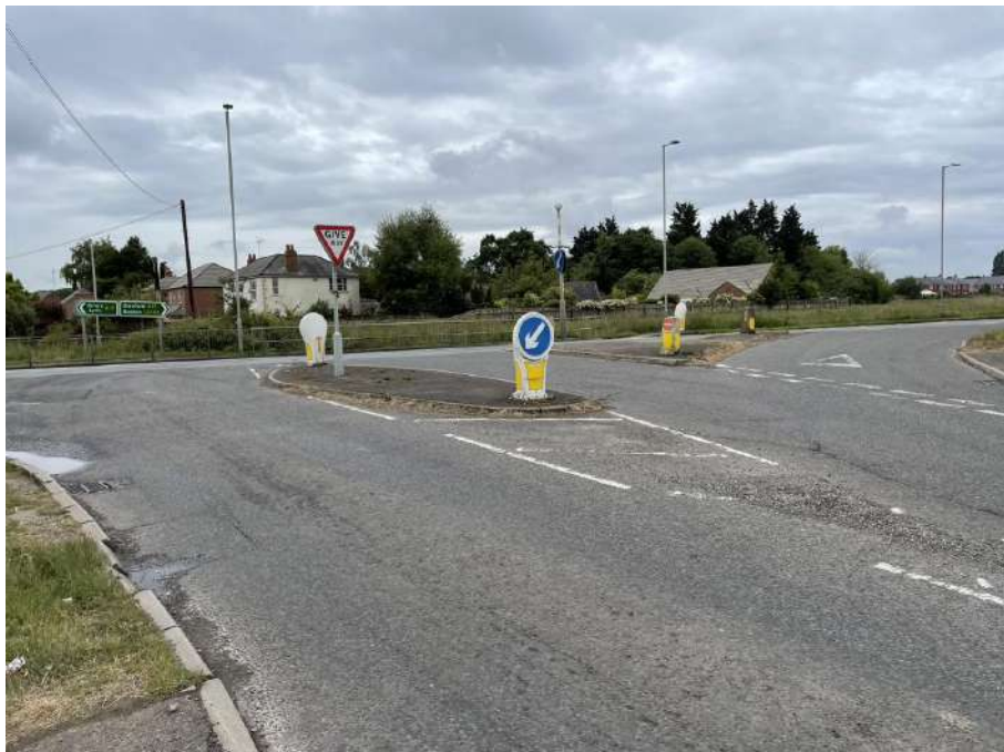
Photo 3: A17/Lowgate Priority Junction
