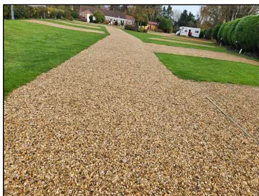
Figure 6 – Gravel access track connecting the road and grassed areas
