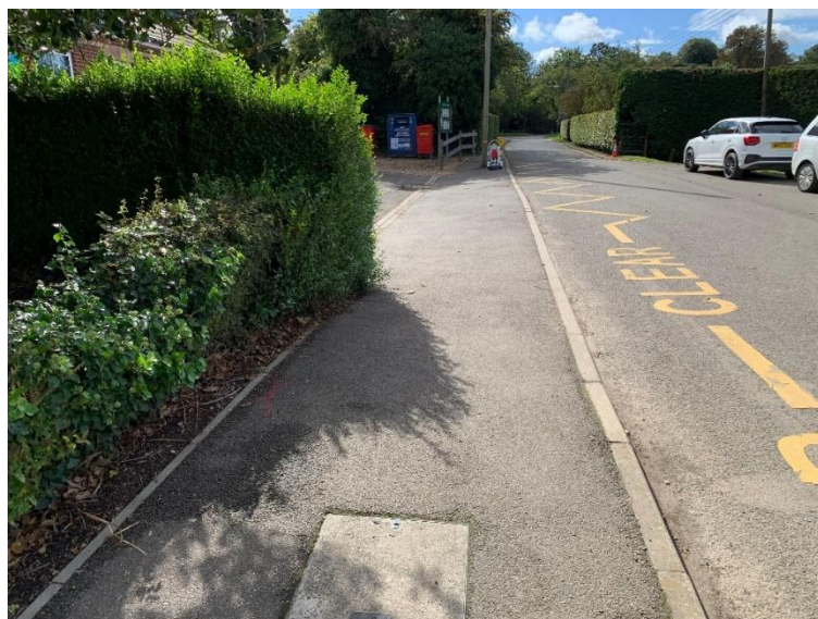
Photo 3: Footway on Wood Lane
