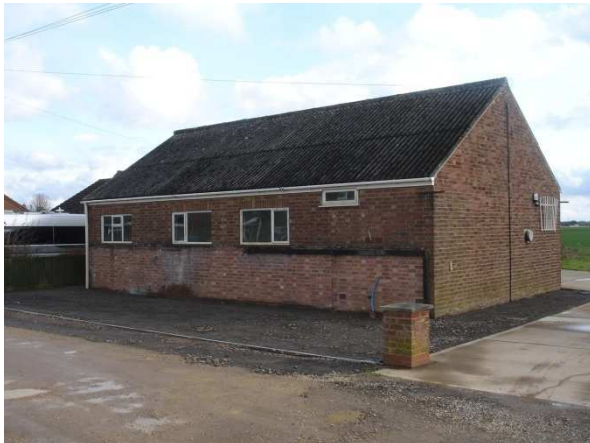
No. 14 outbuilding to the north-east
