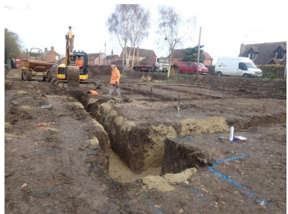
Plate 137: Excavation of the foundations, from the south
