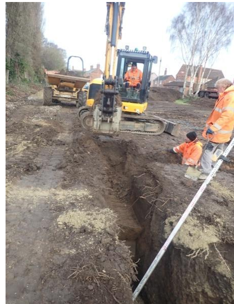
Plate 136: Excavation of the foundations, from the south
