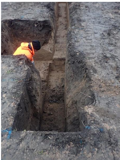
Plate 94: Excavation of the foundations, from the north
