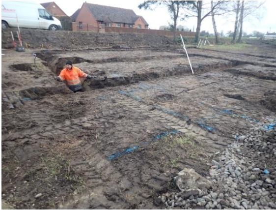
Plate 149: Excavation of the foundations, from the west
