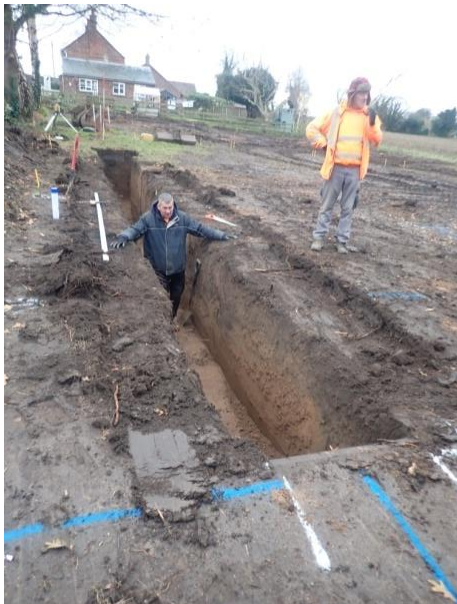
Plate 44: Excavation of the foundations, from the north
