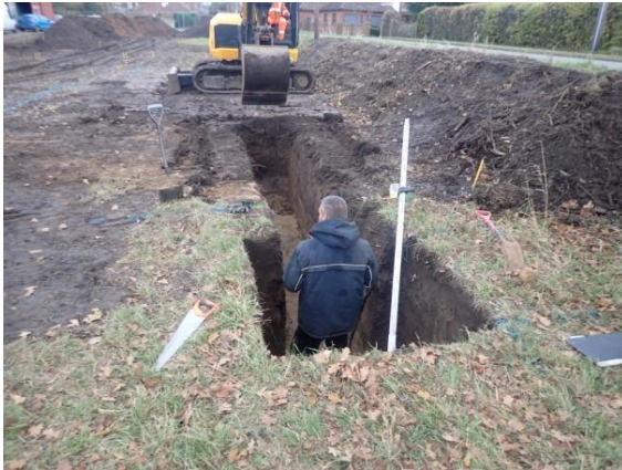
Plate 40: Excavation of the foundations, from the south
