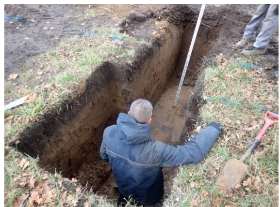
Plate 38: Excavation of the foundations, from the south
