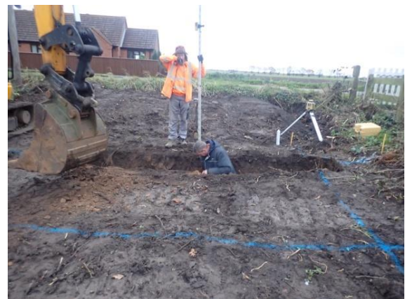
Plate 6: Excavation of the foundations, from the west
