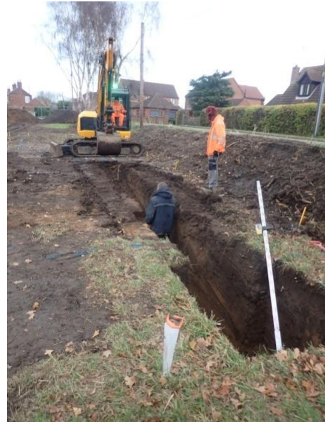
Plate 42: Excavation of the foundations, from the south
