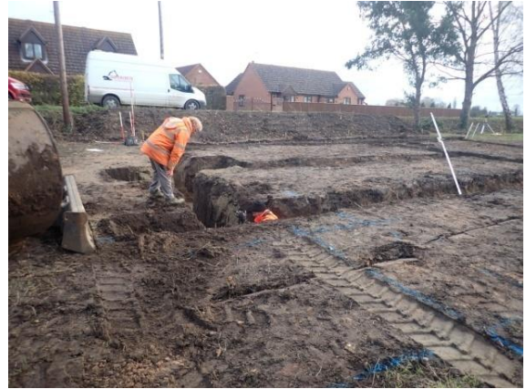
Plate 146: Excavation of the foundations, from the west
