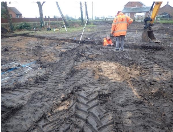
Plate 54: Excavation of the foundations, from the north
