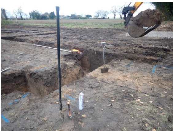
Plate 88: Excavation of the foundations, from the north-east
