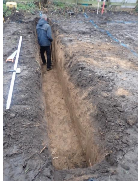
Plate 9: Excavation of the foundations, from the north
