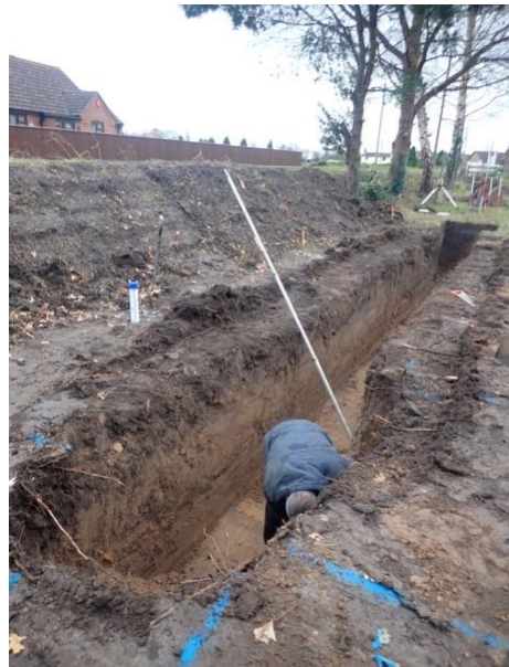
Plate 46: Excavation of the foundations, from the north
