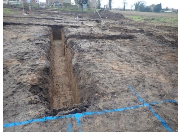
Plate 135: Excavation of the foundations, from the north
