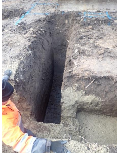
Plate 141: Excavation of the foundations, from the east
