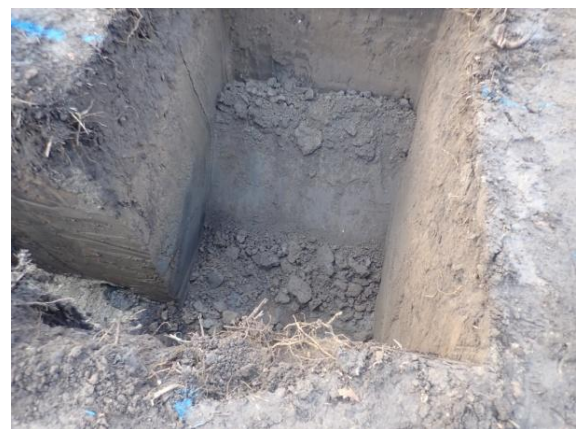
Plate 112: Excavation of the foundations, from the north
