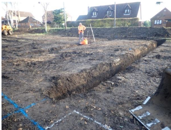
Plate 71: Representative Section 10, from the south-west
