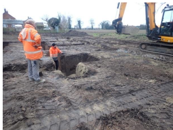
Plate 154: Excavation of the foundations, from the north
