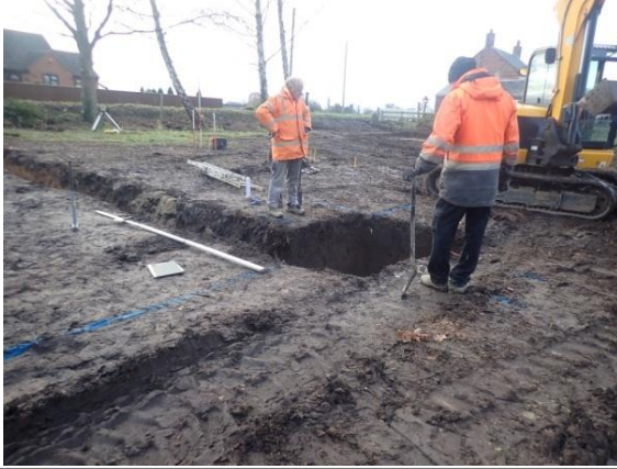
Plate 113: Excavation of the foundations, from the north-west
