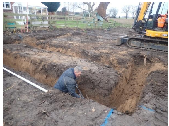
Plate 20: Excavation of the foundations, from the east
