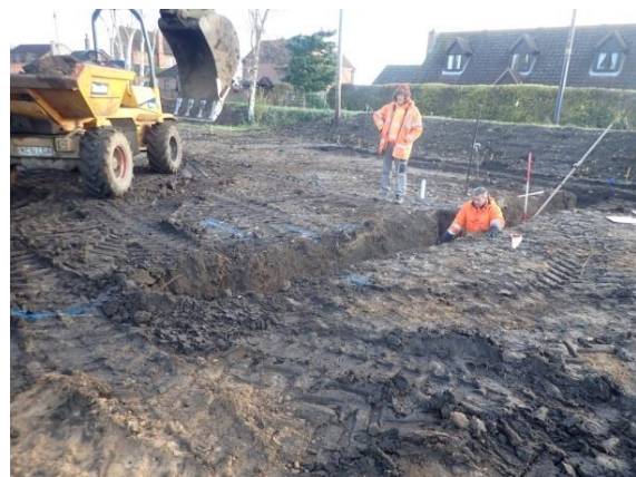
Plate 64: Excavation of the foundations, from the south-west
