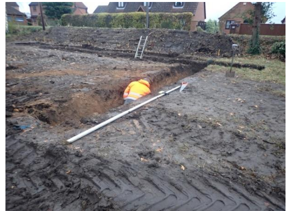
Plate 51: Excavation of the foundations, from the west
