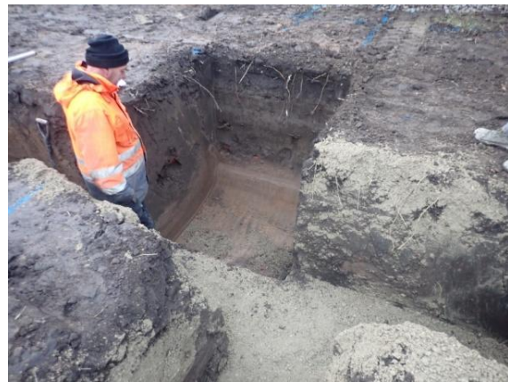
Plate 153: Excavation of the foundations, from the east
