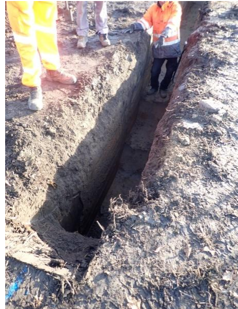
Plate 68: Excavation of the foundations, from the west
