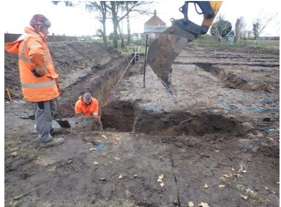
Plate 79: Excavation of the foundations, from the north
