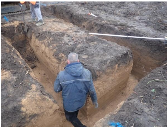
Plate 17: Excavation of the foundations, from the south-west
