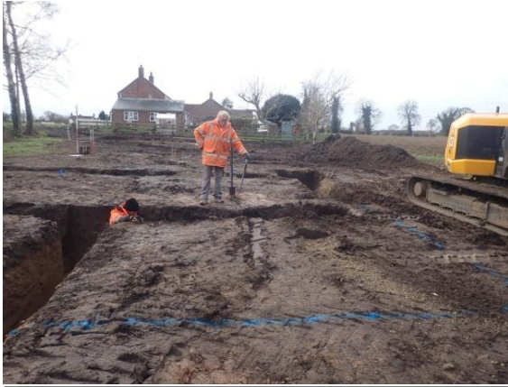
Plate 121: Excavation of the foundations, from the north
