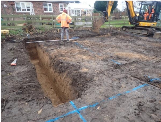
Plate 12: Excavation of the foundations, from the north
