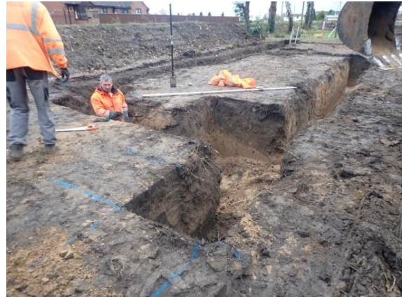
Plate 90: Excavation of the foundations, from the north
