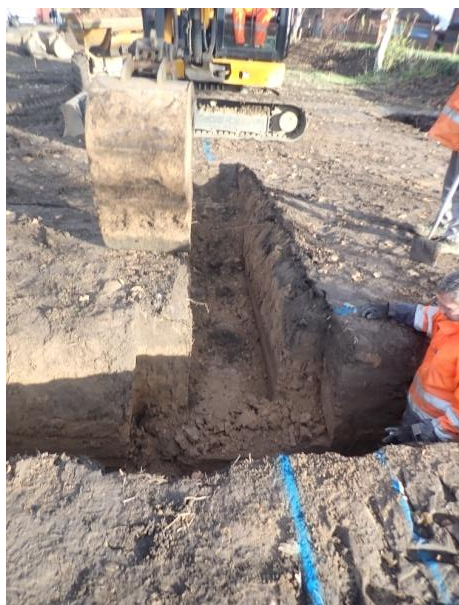
Plate 72: Excavation of the foundations, from the south
