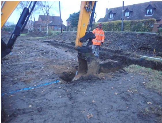
Plate 48: Excavation of the foundations, from the south
