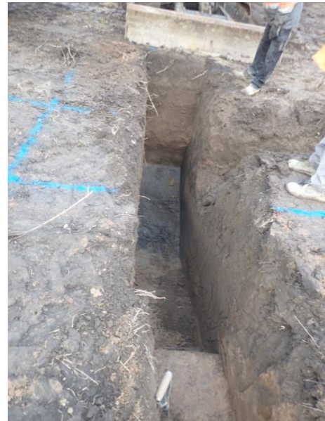
Plate 147: Excavation of the foundations, from the south
