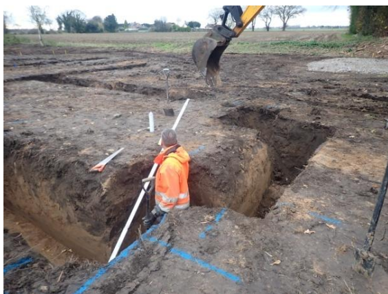
Plate 83: Excavation of the foundations, from the east
