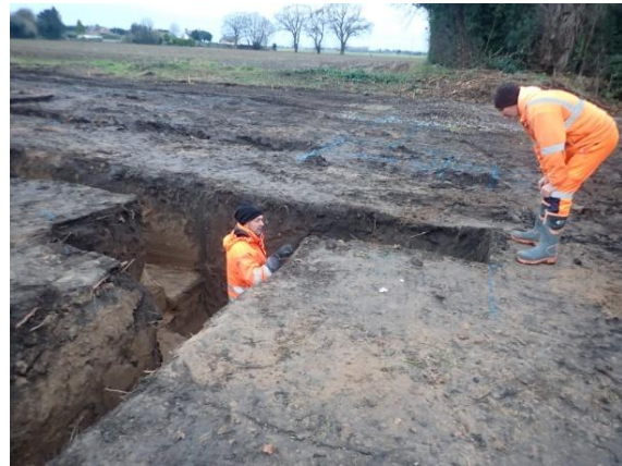
Plate 96: Excavation of the foundations, from the east
