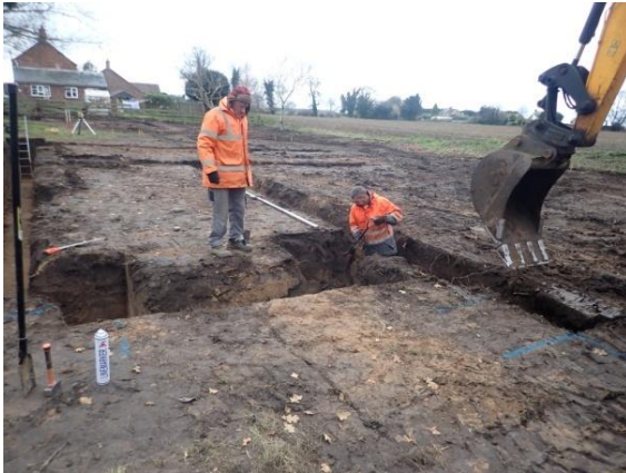
Plate 87: Excavation of the foundations, from the north
