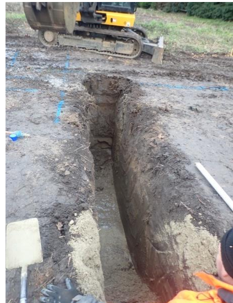
Plate 102: Excavation of the foundations, from the east
