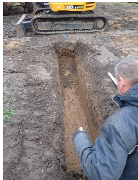
Plate 26: Excavation of the foundations, from the south
