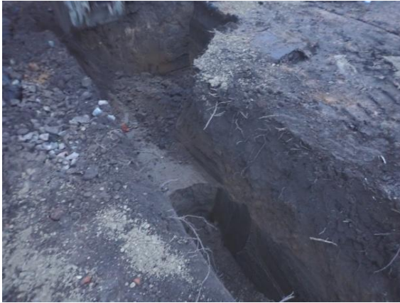
Plate 161: Excavation of the foundations, from the south
