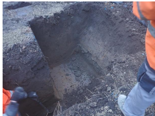
Plate 159: Excavation of the foundations, from the north
