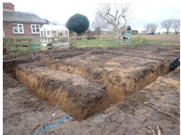
Plate 32: Excavation of the foundations, from the north-east
