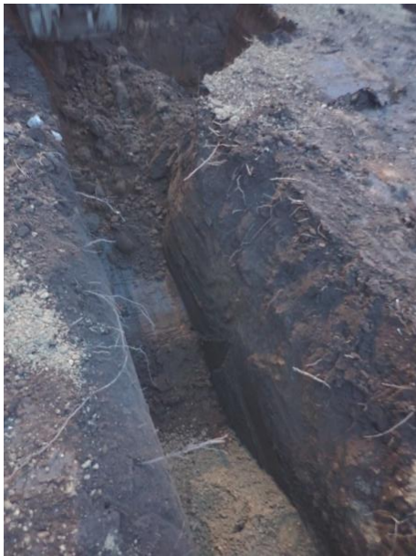
Plate 162: Excavation of the foundations, from the south
