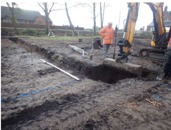
Plate 109: Excavation of the foundations, from the west
