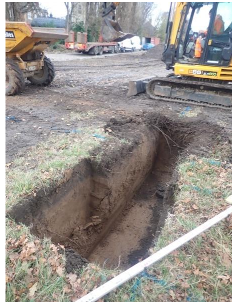
Plate 37: Excavation of the foundations, from the south
