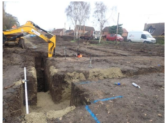
Plate 125: Excavation of the foundations, from the south
