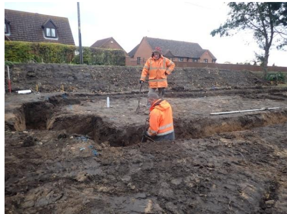
Plate 85: Excavation of the foundations, from the west
