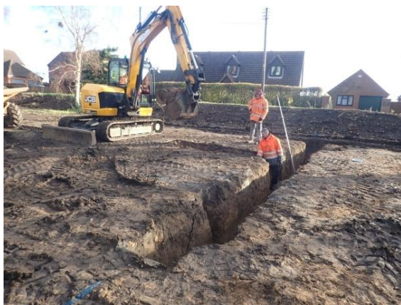
Plate 73: Excavation of the foundations, from the west
