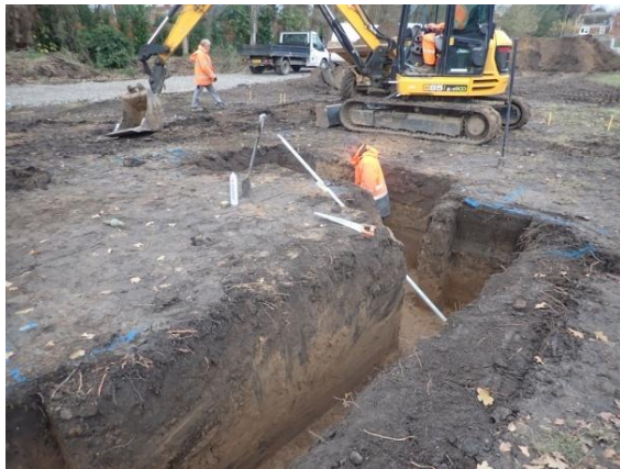
Plate 82: Excavation of the foundations, from the north-east
