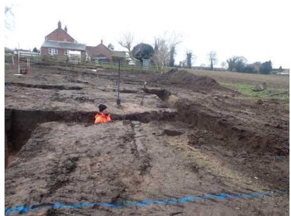
Plate 126: Excavation of the foundations, from the north
