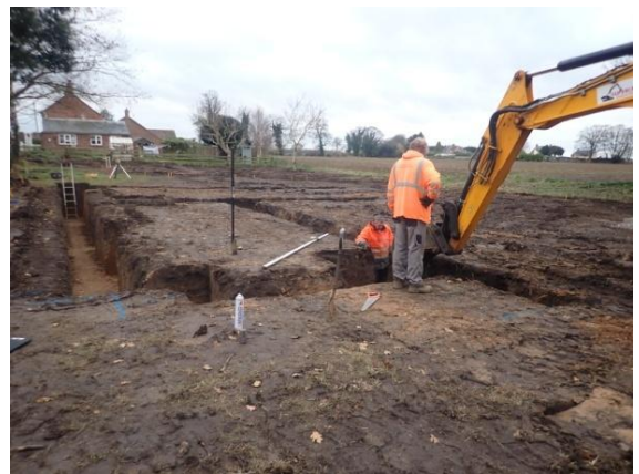
Plate 91: Excavation of the foundations, from the north
