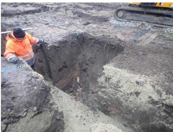
Plate 151: Excavation of the foundations, from the north-east
