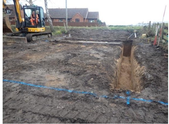
Plate 18: Excavation of the foundations, from the west
