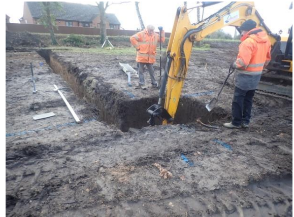
Plate 111: Excavation of the foundations, from the west
