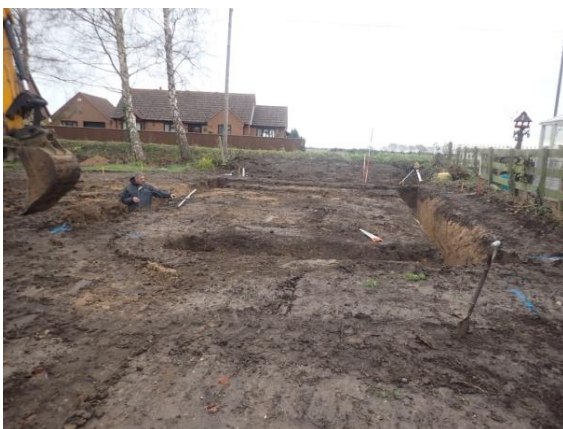
Plate 29: Excavation of the foundations, from the west
