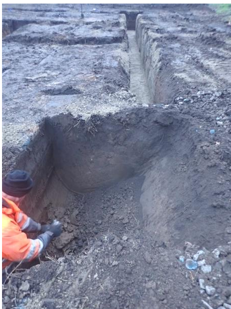
Plate 157: Excavation of the foundations, from the north
