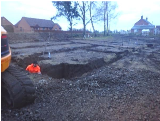
Plate 163: Excavation of the foundations, from the north-west
