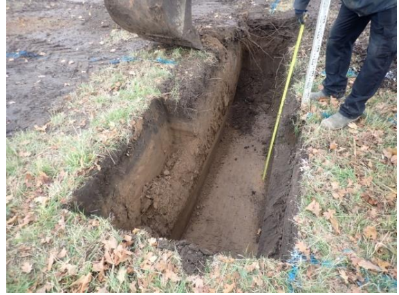
Plate 36: Excavation of the foundations, from the south
