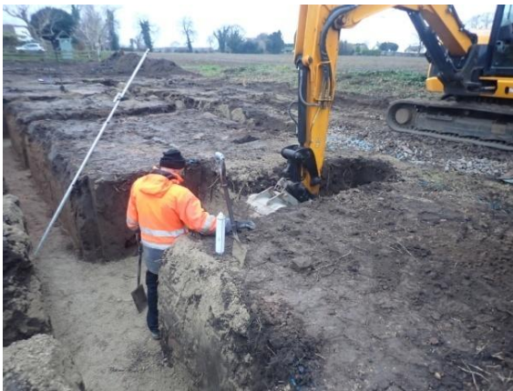
Plate 156: Excavation of the foundations, from the north
