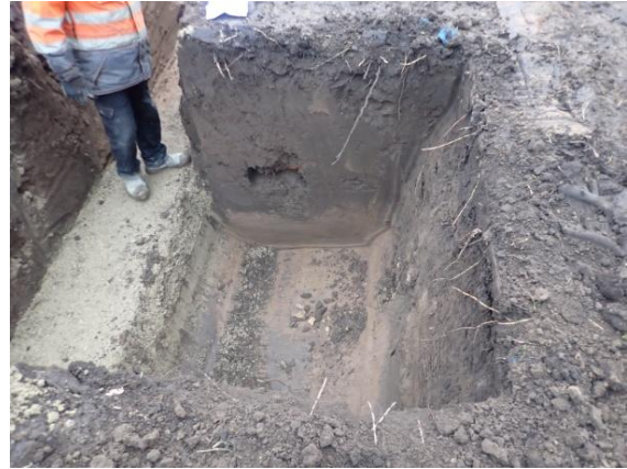
Plate 152: Excavation of the foundations, from the north
