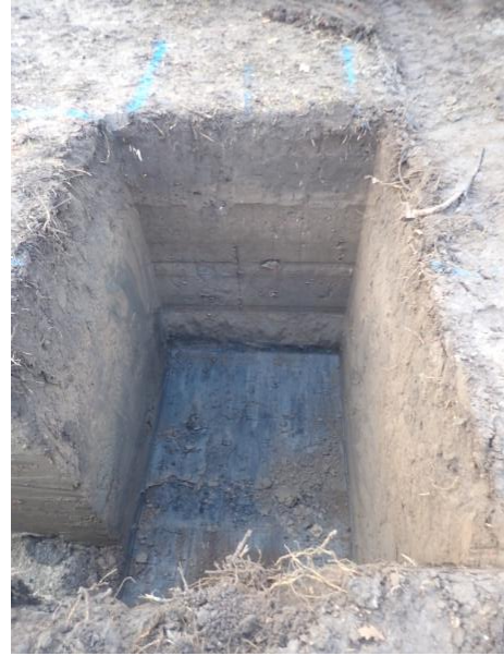
Plate 115: Excavation of the foundations, from the north
