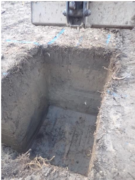
Plate 114: Excavation of the foundations, from the north
