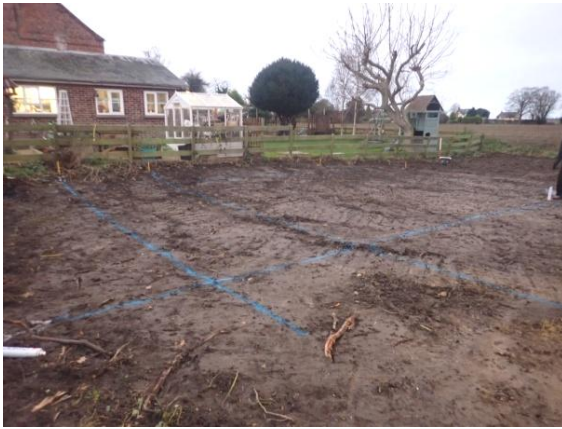
Plate 1: Pre-groundworks, from the north-east
