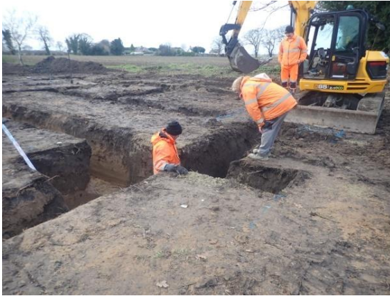
Plate 143: Excavation of the foundations, from the north-east
