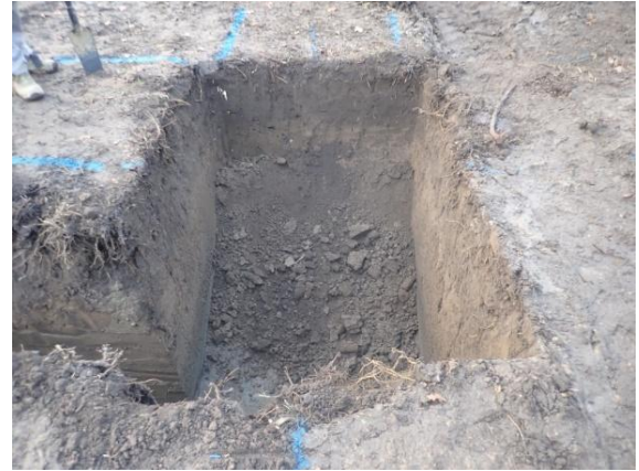
Plate 110: Excavation of the foundations, from the north
