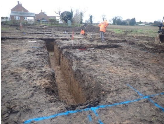
Plate 133: Excavation of the foundations, from the north
