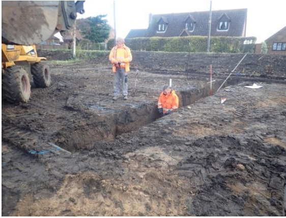
Plate 65: Excavation of the foundations, from the south-west
