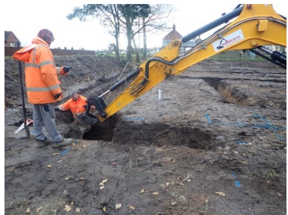
Plate 80: Excavation of the foundations, from the north
