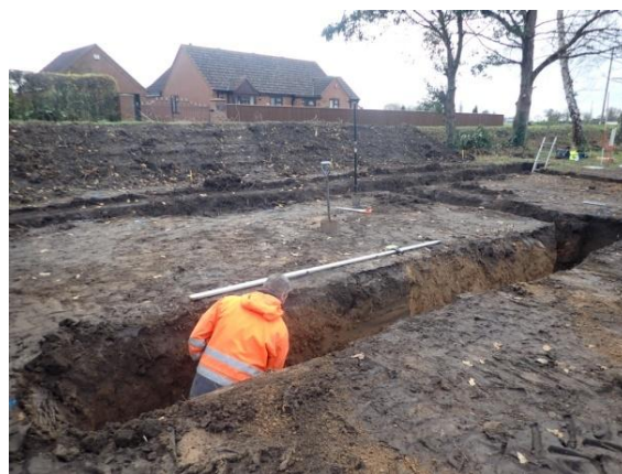
Plate 75: Excavation of the foundations, from the north-west
