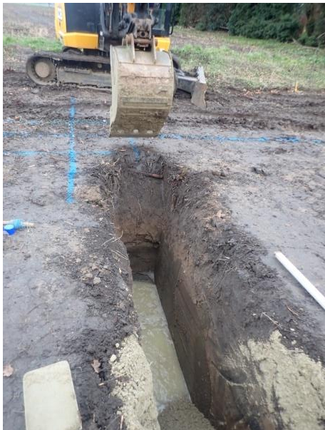
Plate 99: Excavation of the foundations, from the east
