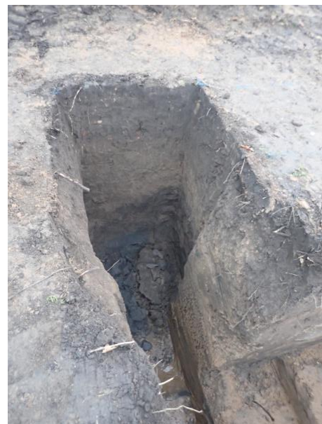
Plate 97: Excavation of the foundations, from the south
