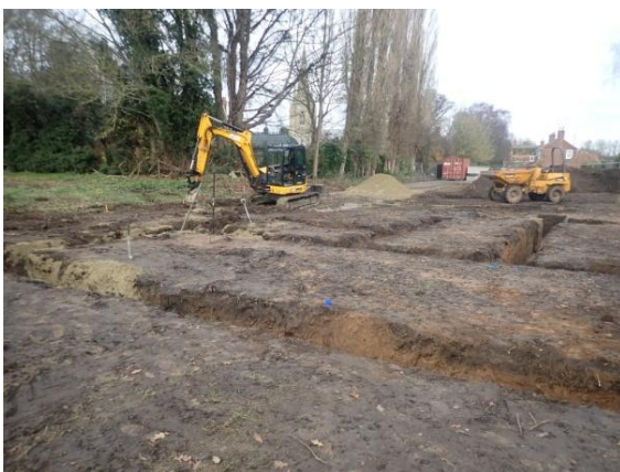
Plate 134: Excavation of the foundations, from the south
