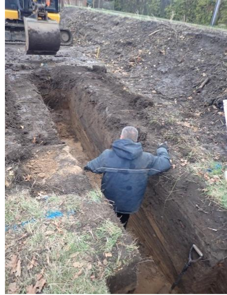
Plate 41: Excavation of the foundations, from the south
