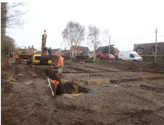
Plate 123: Excavation of the foundations, from the south
