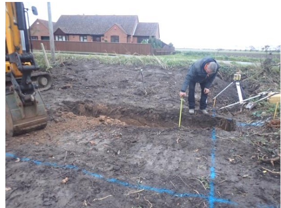
Plate 5: Excavation of the foundations, from the west
