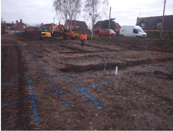
Plate 92: Excavation of the foundations, from the south
