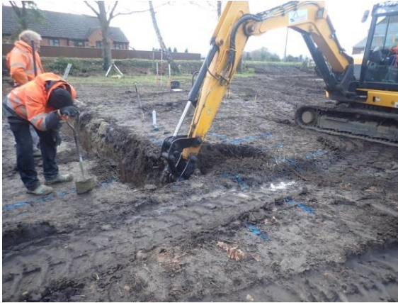
Plate 107: Excavation of the foundations, from the west
