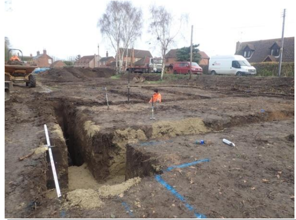
Plate 124: Excavation of the foundations, from the south
