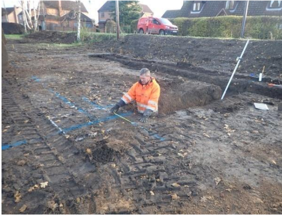
Plate 59: Excavation of the foundations, from the south
