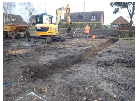
Plate 58: Excavation of the foundations, from the south-west
