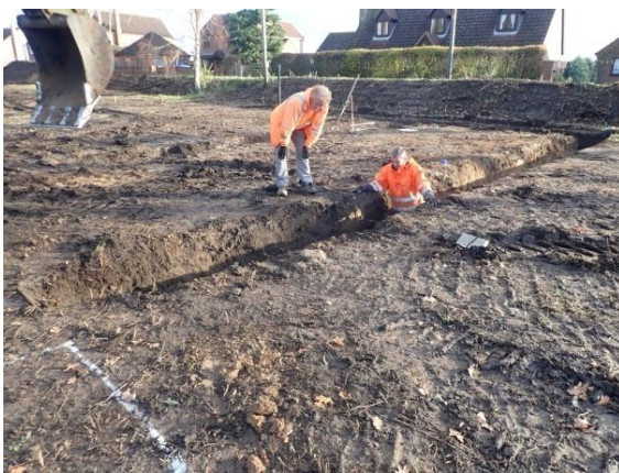
Plate 67: Excavation of the foundations, from the south-west
