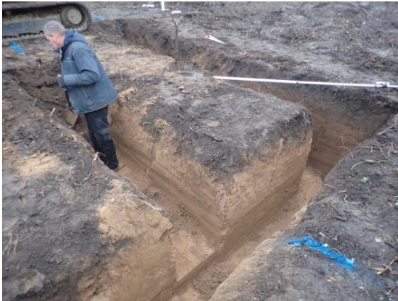
Plate 16: Excavation of the foundations, from the south-west
