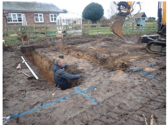
Plate 19: Excavation of the foundations, from the north
