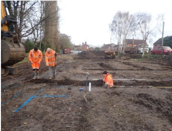
Plate 104: Excavation of the foundations, from the south
