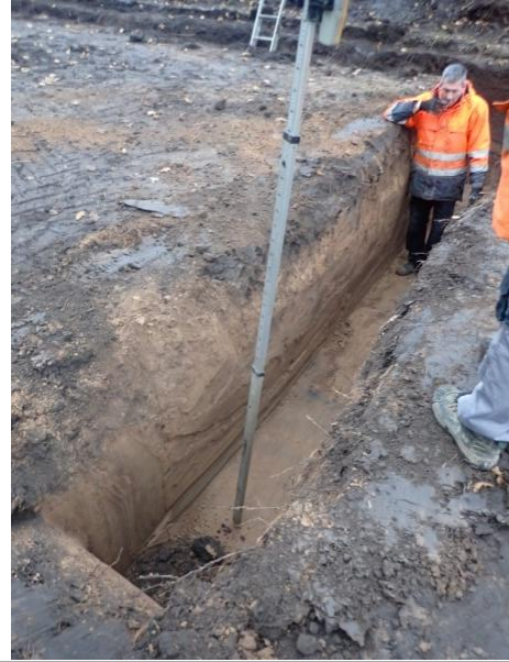
Plate 50: Excavation of the foundations, from the west
