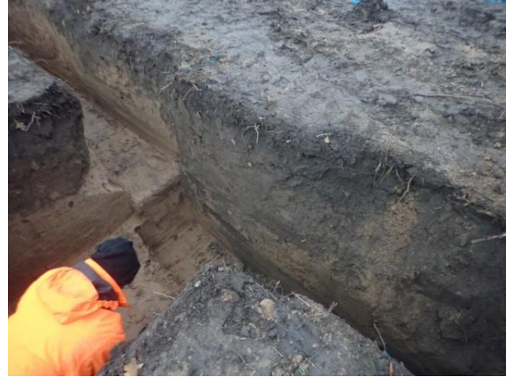
Plate 95: Excavation of the foundations, from the north-east
