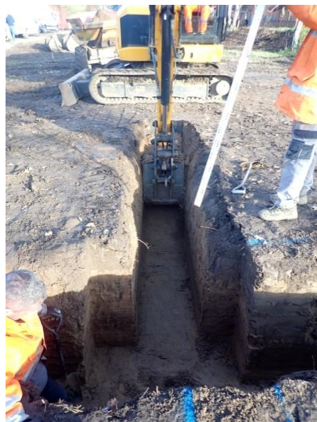
Plate 74: Excavation of the foundations, from the south
