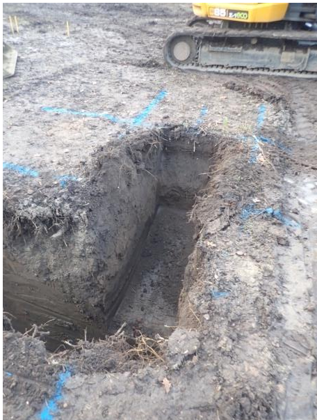
Plate 108: Excavation of the foundations, from the west
