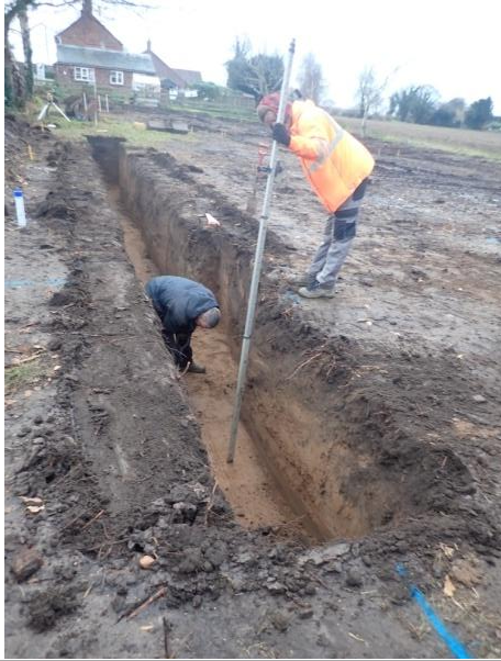
Plate 47: Excavation of the foundations, from the north
