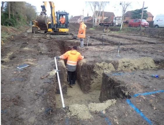
Plate 122: Excavation of the foundations, from the south
