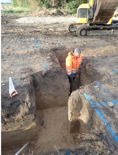
Plate 81: Excavation of the foundations, from the east
