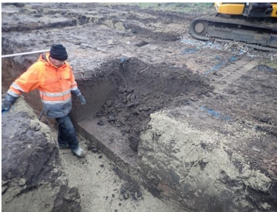
Plate 150: Excavation of the foundations, from the north-east
