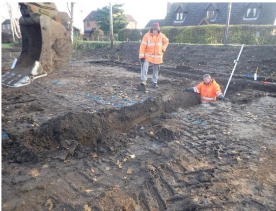
Plate 60: Excavation of the foundations, from the south-west
