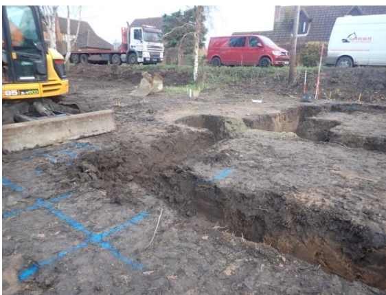
Plate 145: Excavation of the foundations, from the south-east
