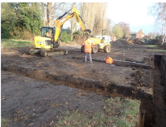
Plate 61: Excavation of the foundations, from the south
