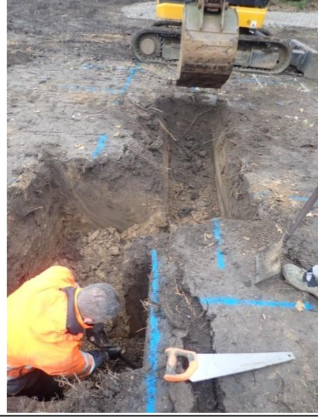
Plate 78: Excavation of the foundations, from the east
