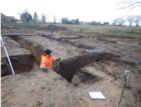
Plate 144: Excavation of the foundations, from the north-east
