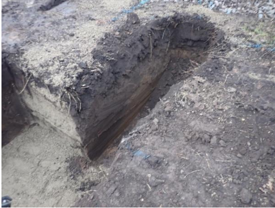
Plate 155: Excavation of the foundations, from the north-east
