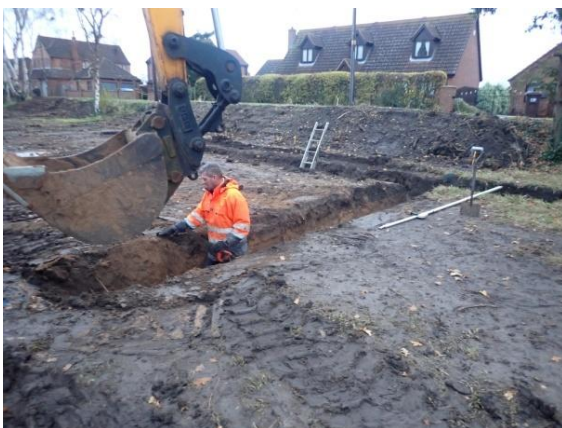
Plate 49: Excavation of the foundations, from the south-west
