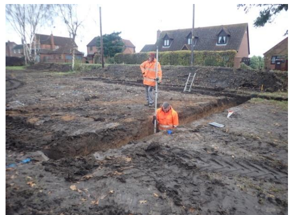
Plate 52: Excavation of the foundations, from the south-west
