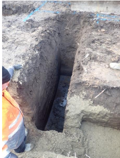
Plate 142: Excavation of the foundations, from the east
