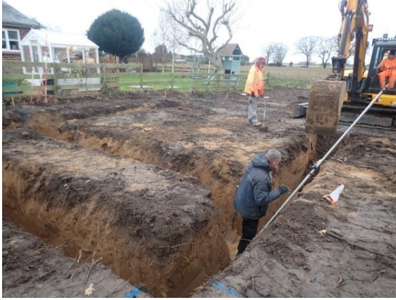
Plate 21: Excavation of the foundations, from the east
