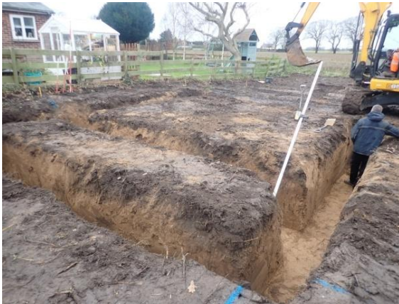
Plate 22: Excavation of the foundations, from the east
