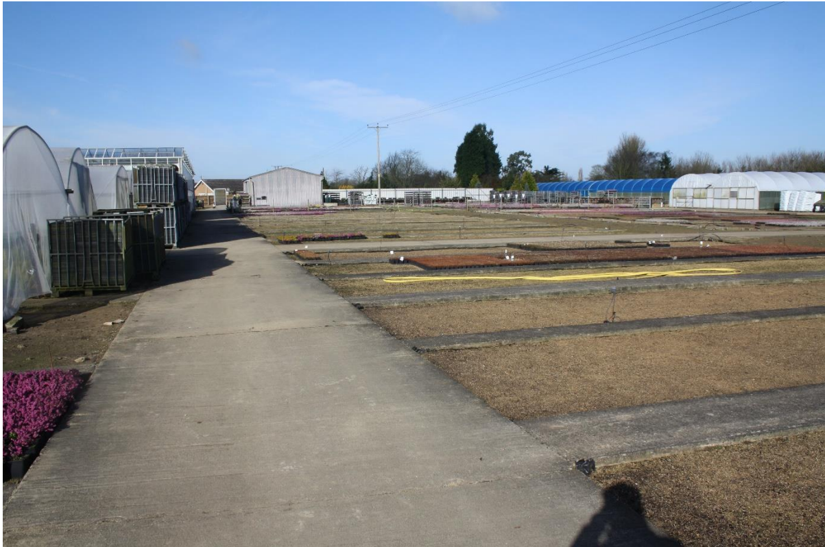
View looking west to the proposed site of building
