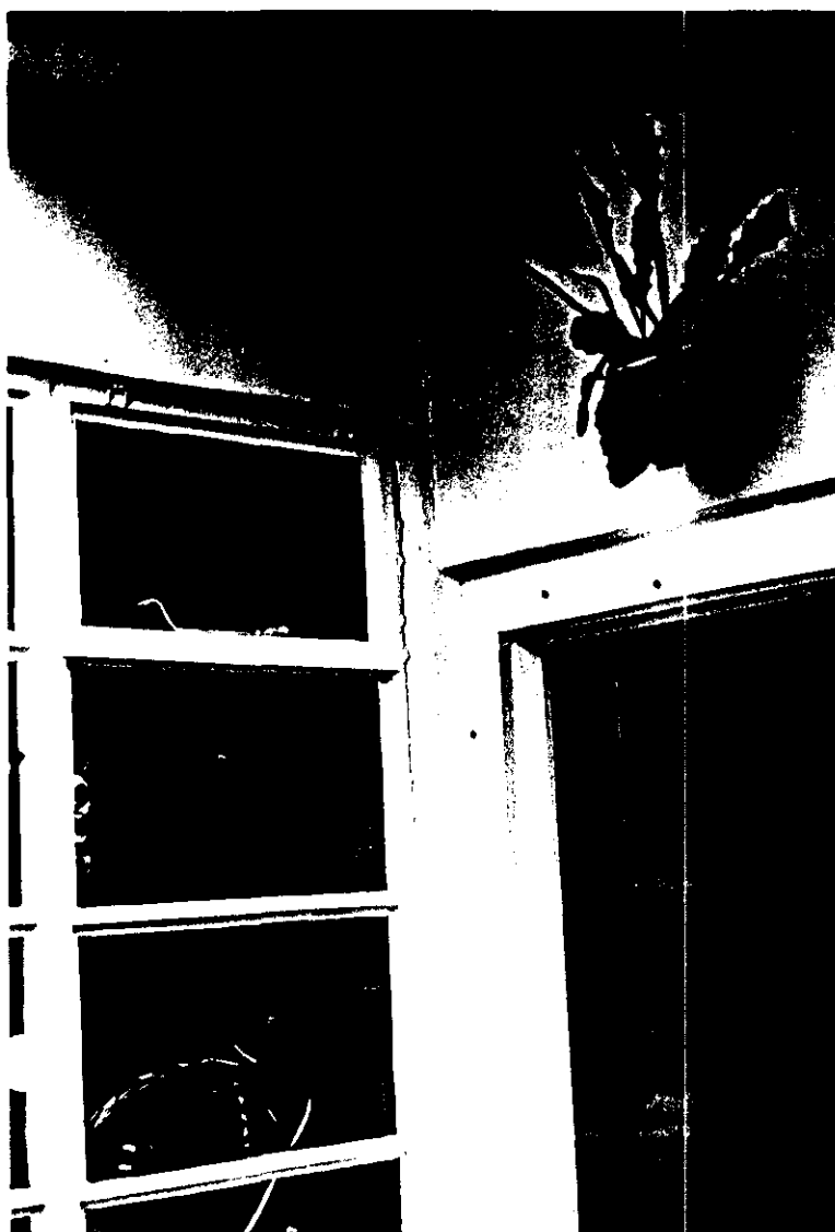
CONSERVATORY WEST WALL. VERTICAL CRACK OVER DOOR OPENING, HORIZONTAL CRACK BETWEEN
