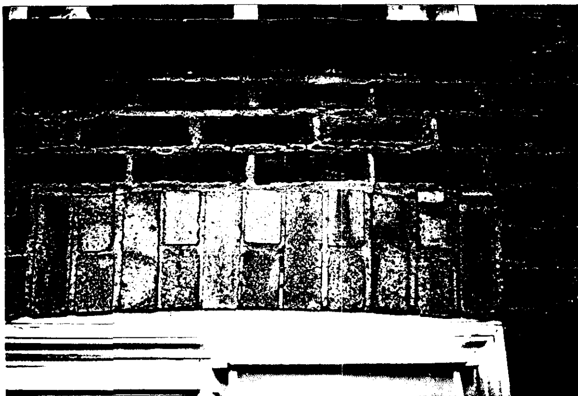
NORTH ELEVATION (REAR) CRACKING ABOVE STUDY WINDOW
