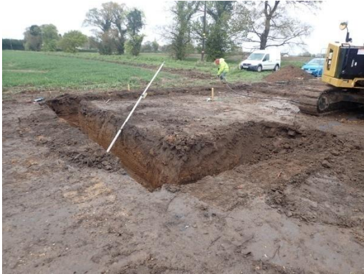
Plate 13: Excavation of the foundations, from the south-west
