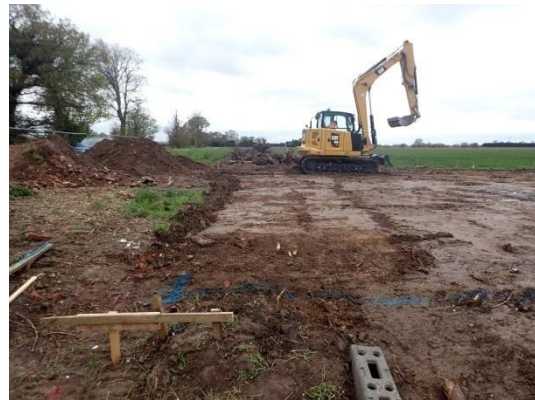
Plate 5: Initial ground reduction, from the north
