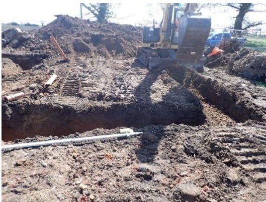
Plate 39: Excavation of the foundations, from the west
