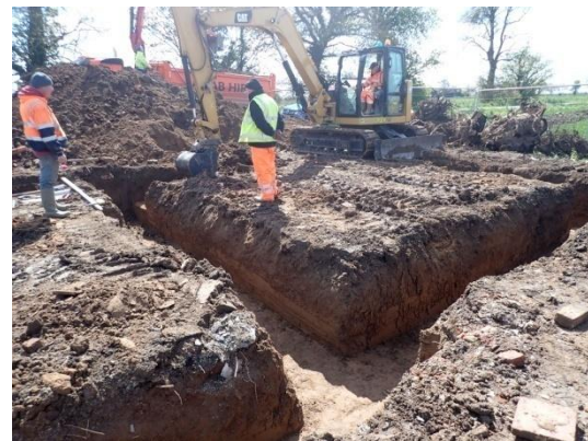
Plate 42: Excavation of the foundations, from the north-west
