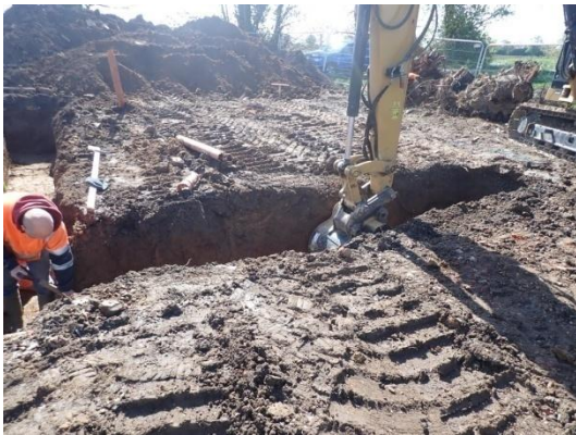
Plate 38: Excavation of the foundations, from the west
