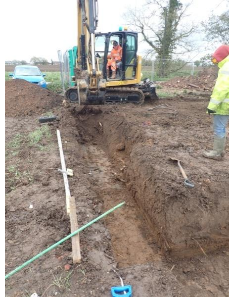
Plate 22: Excavation of the foundations, from the west
