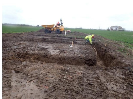
Plate 16: Excavation of the foundations, from the east
