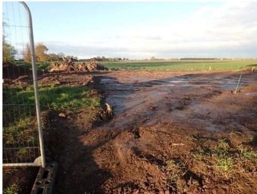
Plate 2: Pre-groundworks, from the north
