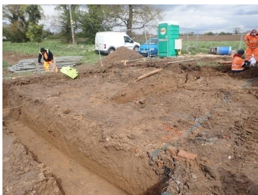
Plate 26: Excavation of the foundations, from the south-west
