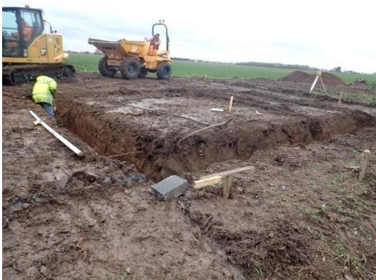
Plate 21: Excavation of the foundations, from the north-west
