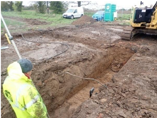
Plate 20: Excavation of the foundations, from the south-west
