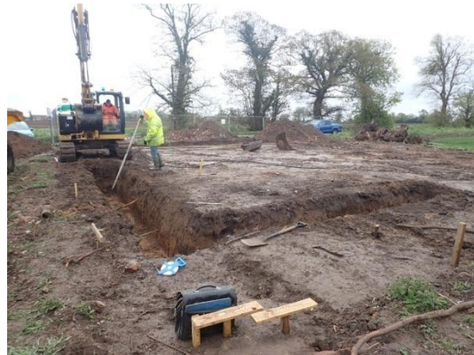
Plate 11: Excavation of the foundations, from the west
