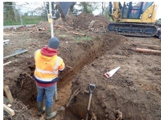
Plate 24: Excavation of the foundations, from the north
