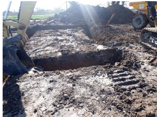
Plate 35: Excavation of the foundations, from the west
