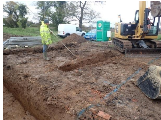
Plate 23: Excavation of the foundations, from the south-west
