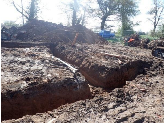
Plate 37: Excavation of the foundations, from the north-west
