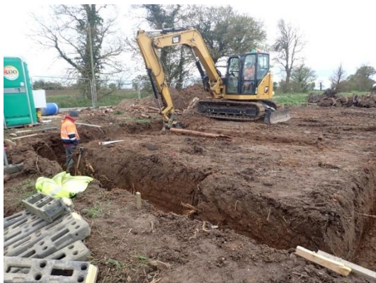
Plate 25: Excavation of the foundations, from the north-west
