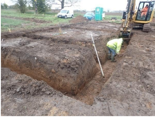
Plate 19: Excavation of the foundations, from the south-west
