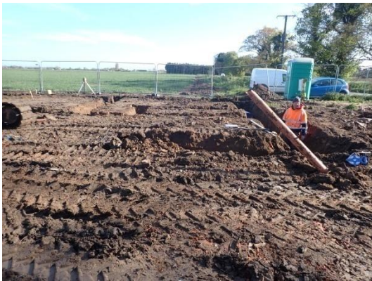
Plate 32: Excavation of the foundations, from the south
