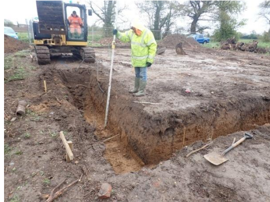
Plate 10: Excavation of the foundations, from the west
