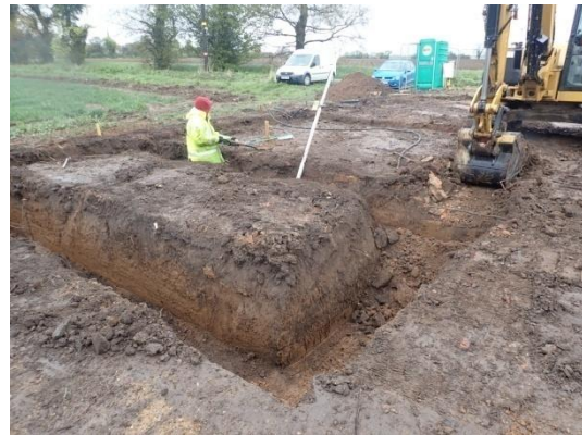
Plate 17: Excavation of the foundations, from the south-west
