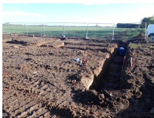
Plate 30: Excavation of the foundations, from the south
