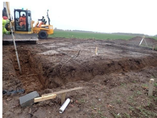
Plate 12: Excavation of the foundations, from the north
