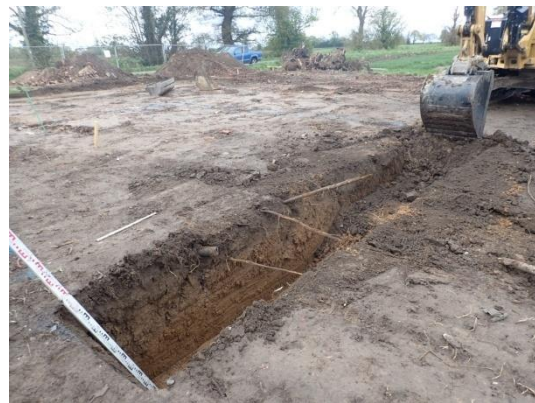
Plate 6: Excavation of the foundations, from the north-west
