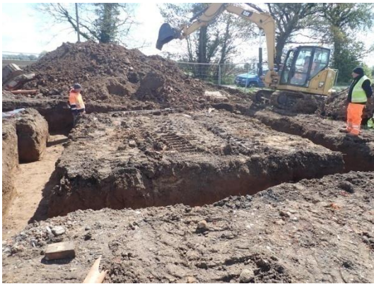
Plate 44: Excavation of the foundations, from the west
