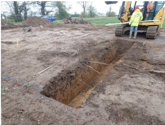
Plate 8: Excavation of the foundations, from the north-west
