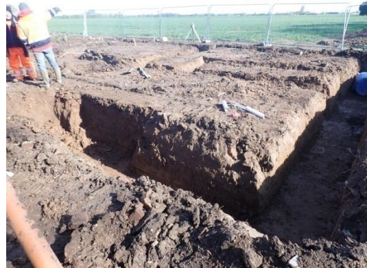
Plate 34: Excavation of the foundations, from the south-east
