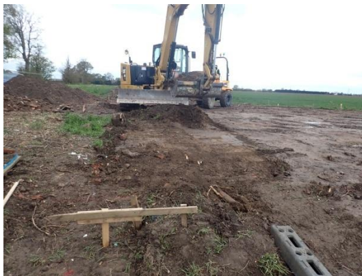
Plate 3: Initial ground reduction, from the north
