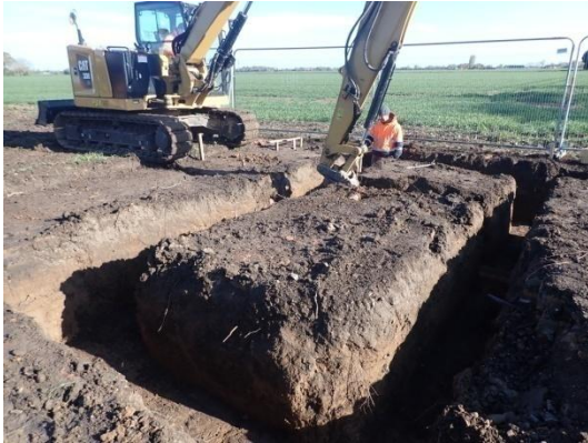
Plate 31: Excavation of the foundations, from the south-east
