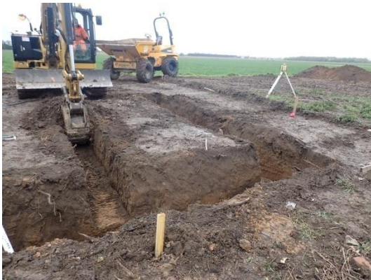
Plate 14: Excavation of the foundations, from the north
