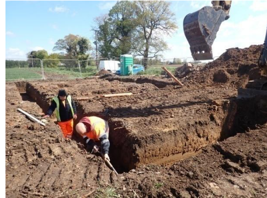
Plate 40: Excavation of the foundations, from the south
