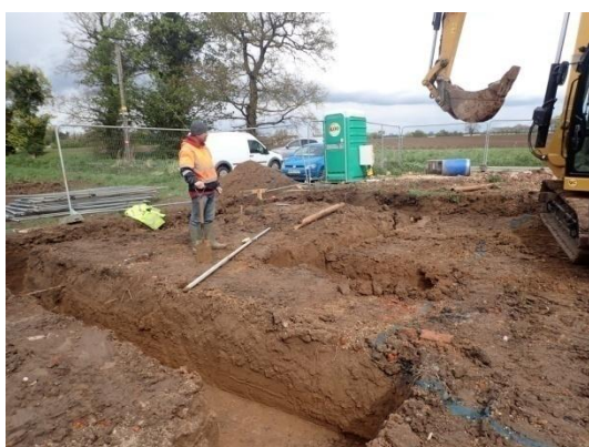
Plate 27: Excavation of the foundations, from the south-west
