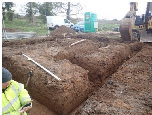
Plate 28: Excavation of the foundations, from the south-west
