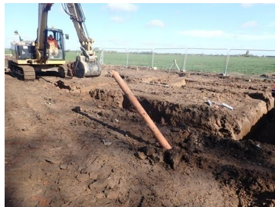
Plate 36: Excavation of the foundations, from the south-east
