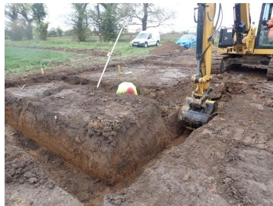
Plate 18: Excavation of the foundations, from the south-west
