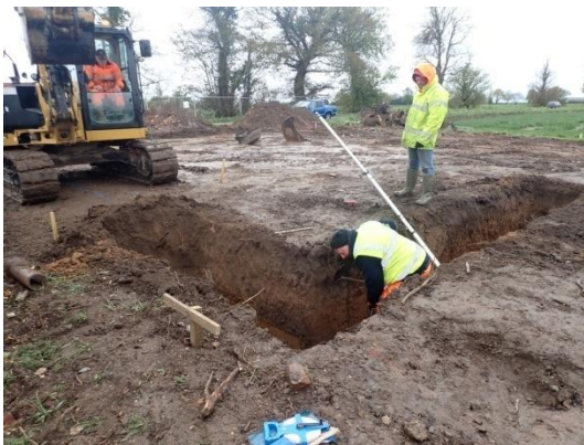
Plate 9: Excavation of the foundations, from the north-west
