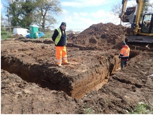
Plate 43: Excavation of the foundations, from the south-west
