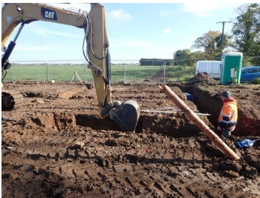
Plate 33: Excavation of the foundations, from the south
