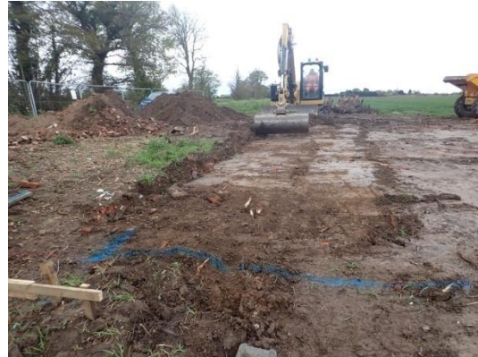
Plate 4: Initial ground reduction, from the north
