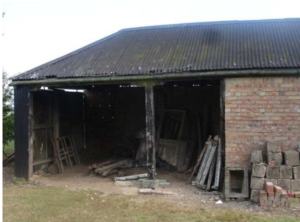
The original cart/implement store opening will become a glazed area serving the living area
