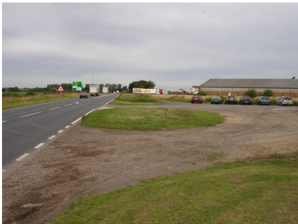
Existing access from A17 Washway Road
