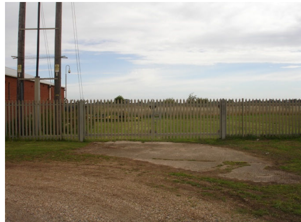
Existing access gates into the grassed compound
