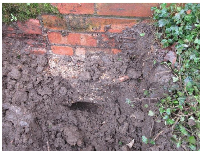
Photograph # 14 (Main 'Stable' Barn - Typical Foundation)
