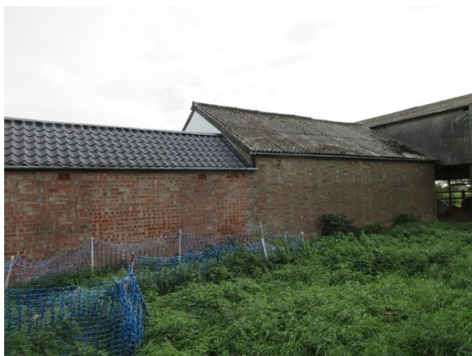
Photograph # 5 (Rear, West Facing Elevation)
