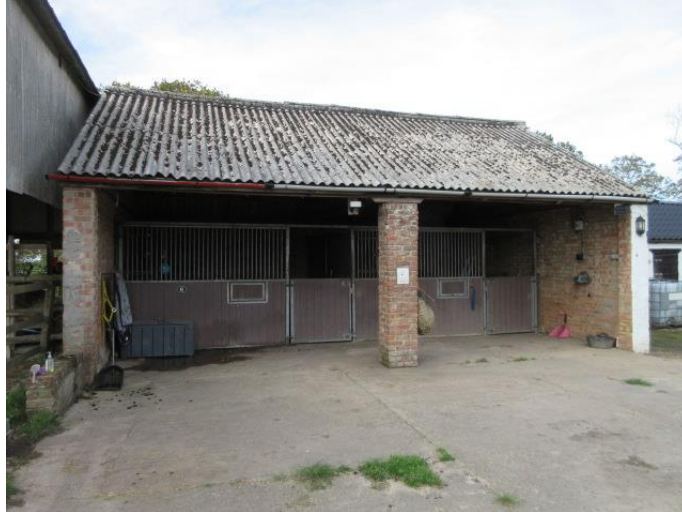
Photograph # 1 (Main 'Stable' Barn - Front, East Facing Elevation)
