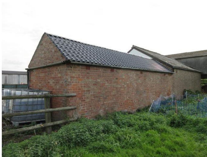
Photograph # 4 ('Store' Barn - North Facing Gable Elevation / West facing Rear Elevation)
