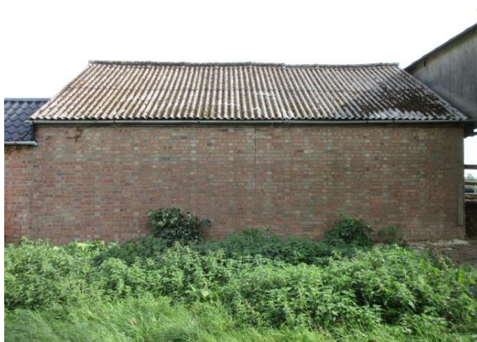
Photograph # 6 (Main 'Stable' Barn - Rear, West Facing Elevation)
