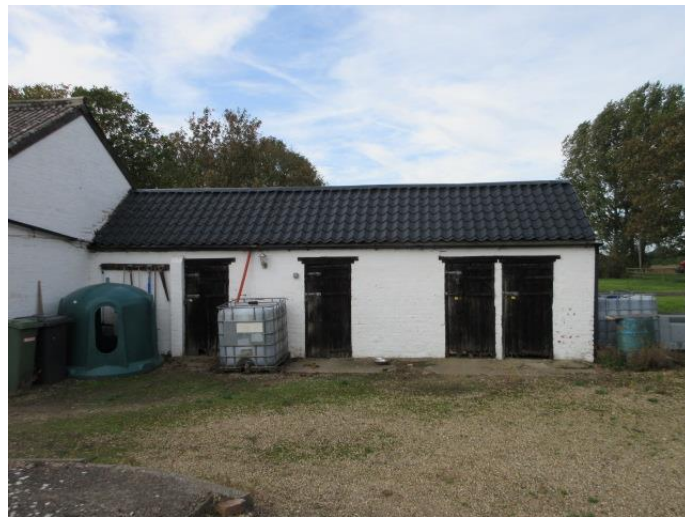
Photograph # 2 ('Store' Barn - Front, East Facing Elevation)
