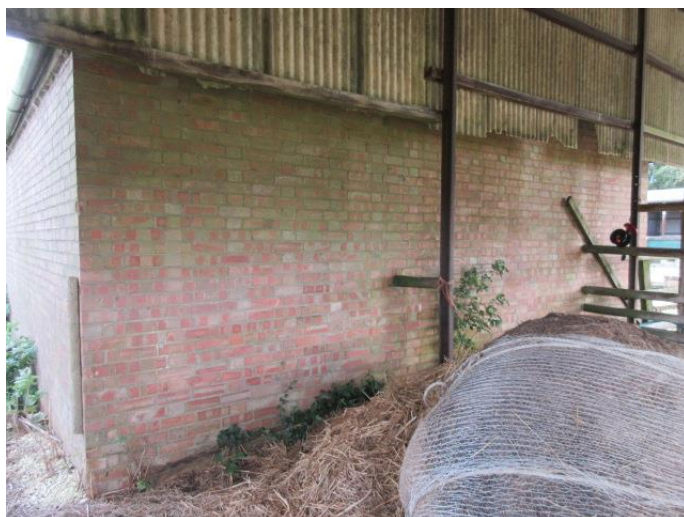
Photograph # 7 (Main 'Stable' Barn - Gable, South Facing Elevation)
