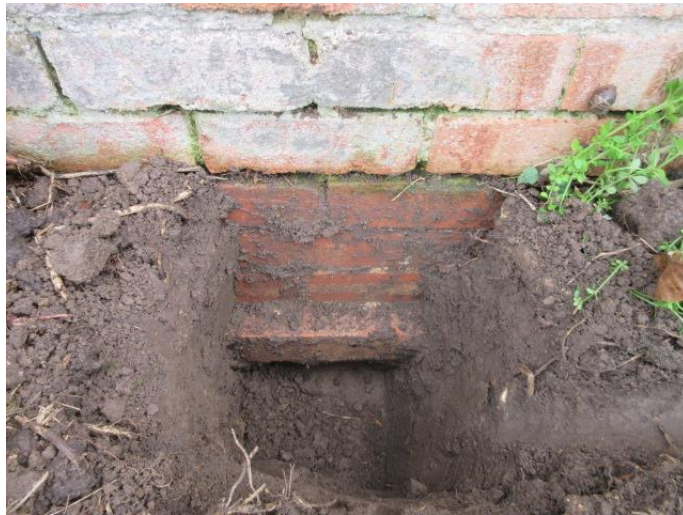
Photograph # 17 ('Store' Barn - Typical Foundation)
