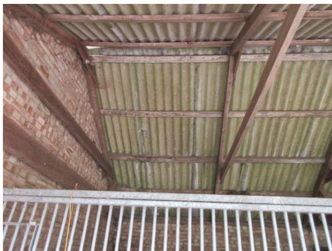
Photograph # 10 (Typical Roof)
