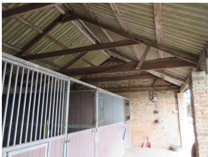
Photograph # 9 (Typical Roof / Eaves Timber Beam onto Central Pier)
