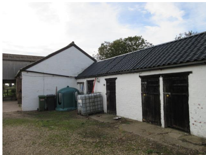
Photograph # 3 (Main 'Stable' Barn North Facing Gable Elevation)
