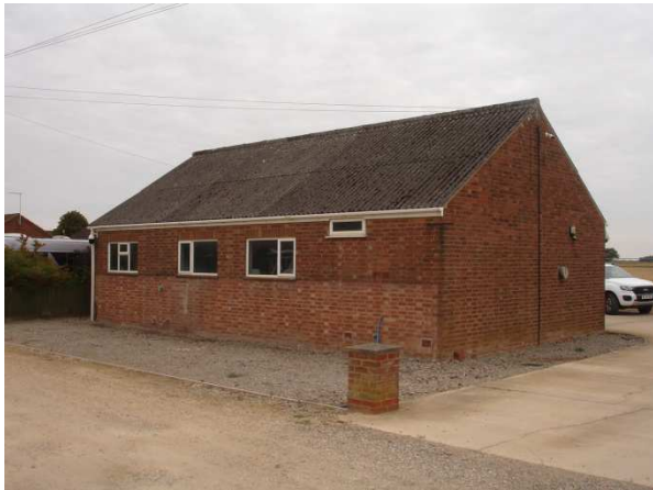
No. 14 outbuilding to the north-east
