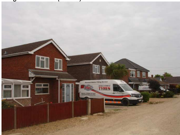
Houses opposite to north (no.s 9, 11 & 13)
