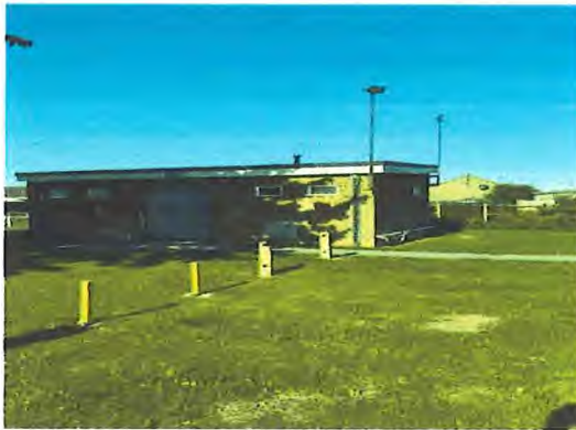
Right hand side of Pavillion – area for container
