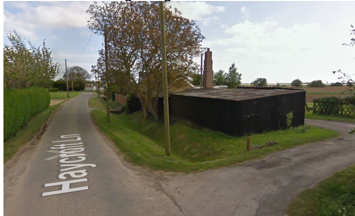
Photo showing a few remaining outbuildings before applicant demolished.
