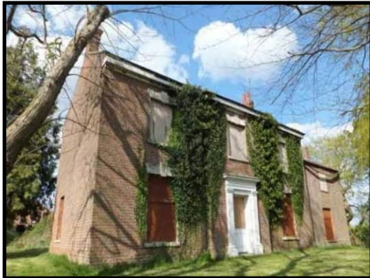
Typical Georgian exterior of the dwelling dating from around 1820
