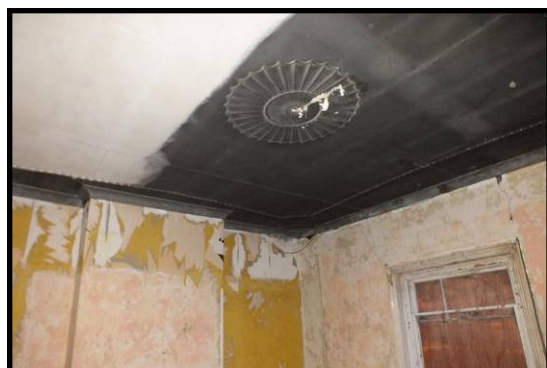
Original plaster mouldings to the ceiling of a first floor bedroom
