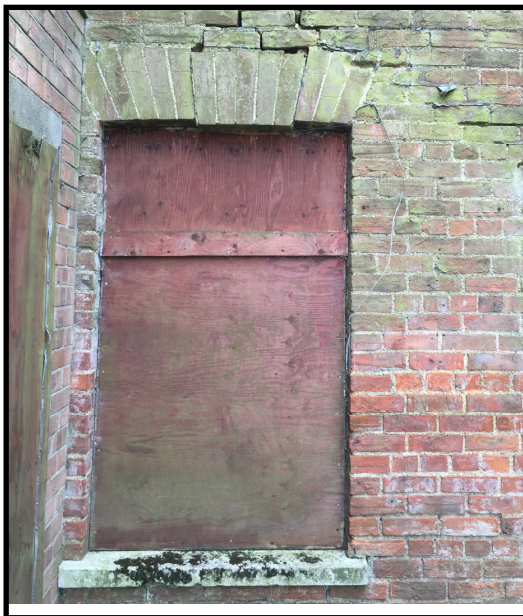
Examples of where brick arches over openings have slipped and caused damage
