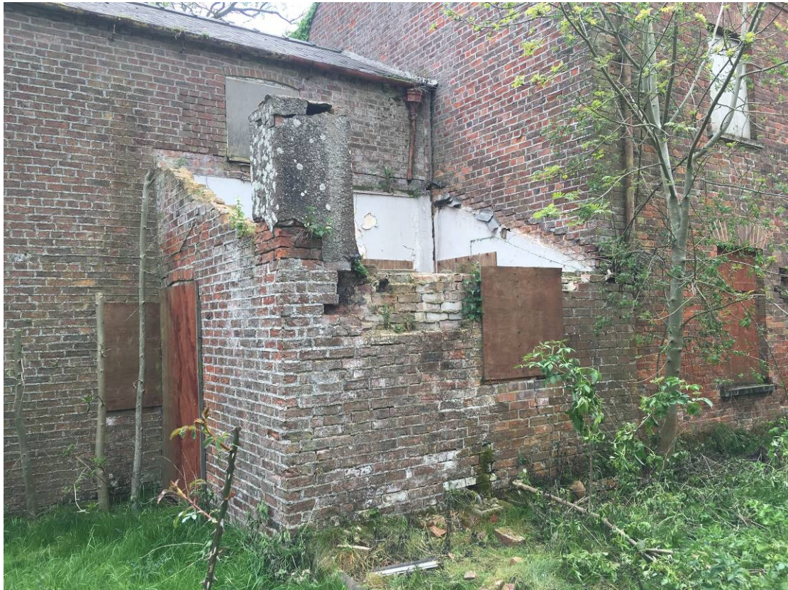
Annex kitchen to the rear that requires demolition and re-building
