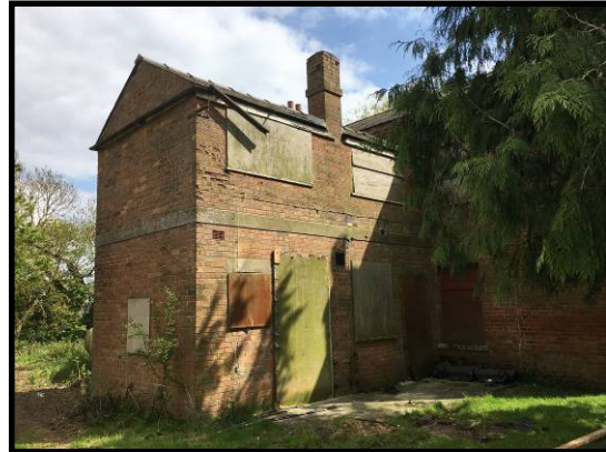
Later unsympathetic extension to the rear of the dwelling
