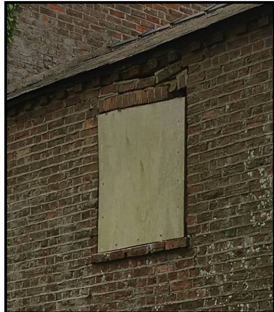
Examples of where brick arches over openings have slipped and caused damage
