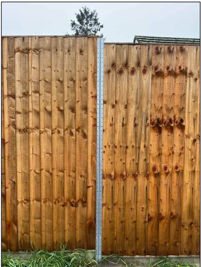
DURAPOST SUPPORT INSTALLATION BEFORE CLADDING APPLIED N.T.S.
