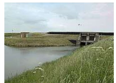
Lawyers Sluice, built in 1949, with the 2003 pumping station to the left
