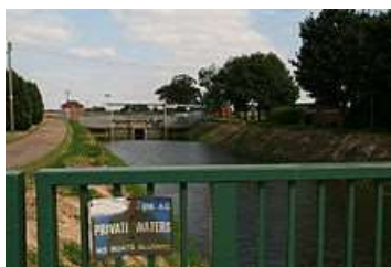
Wiseman's Sluice and Pumping Station on the South Holland Main Drain
