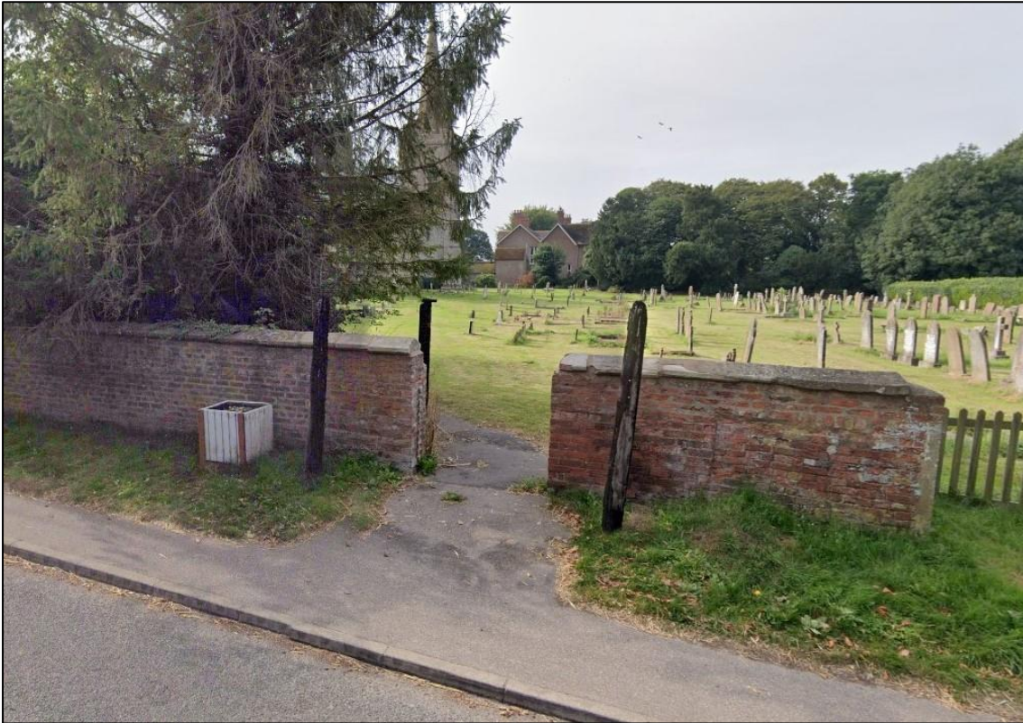
The destroyed Lych Gate c2021
