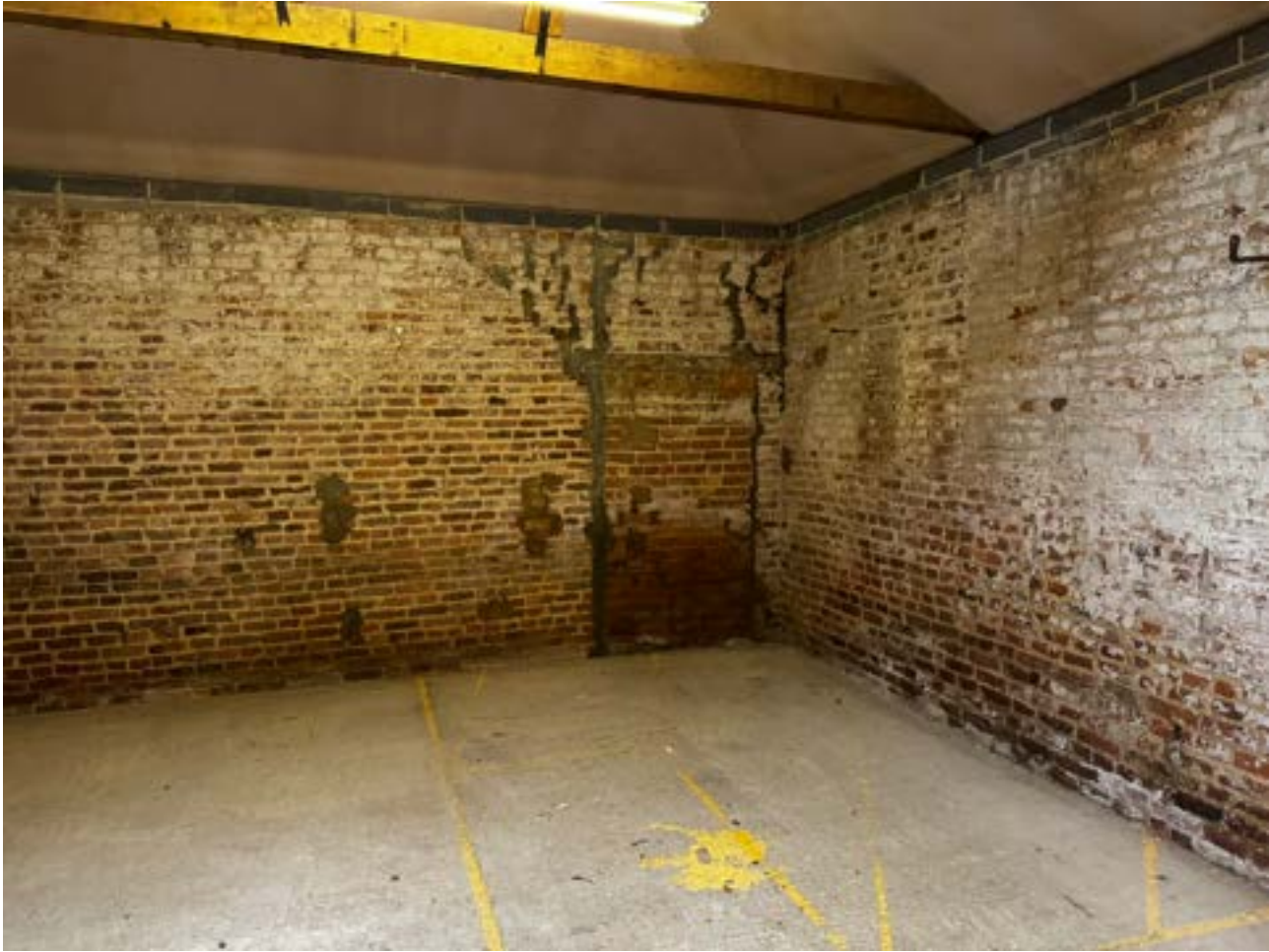
Image 7.0: View of barn structure with concrete floor
