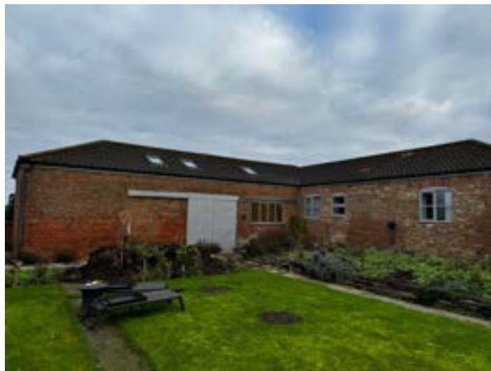
Image 1.0: external view of Barn structure
