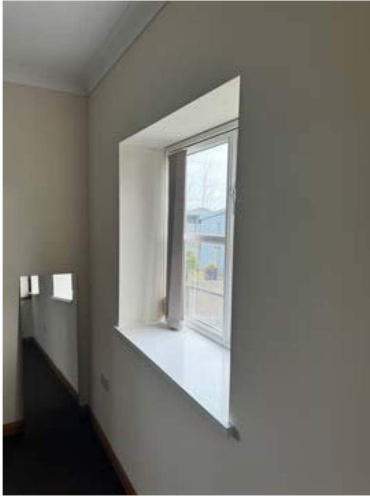
Image 4.0: Deep walls to converted section of barn.
