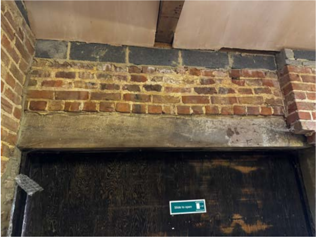
Image 8.0: Timber lintel set to head of sliding door opening into barn
