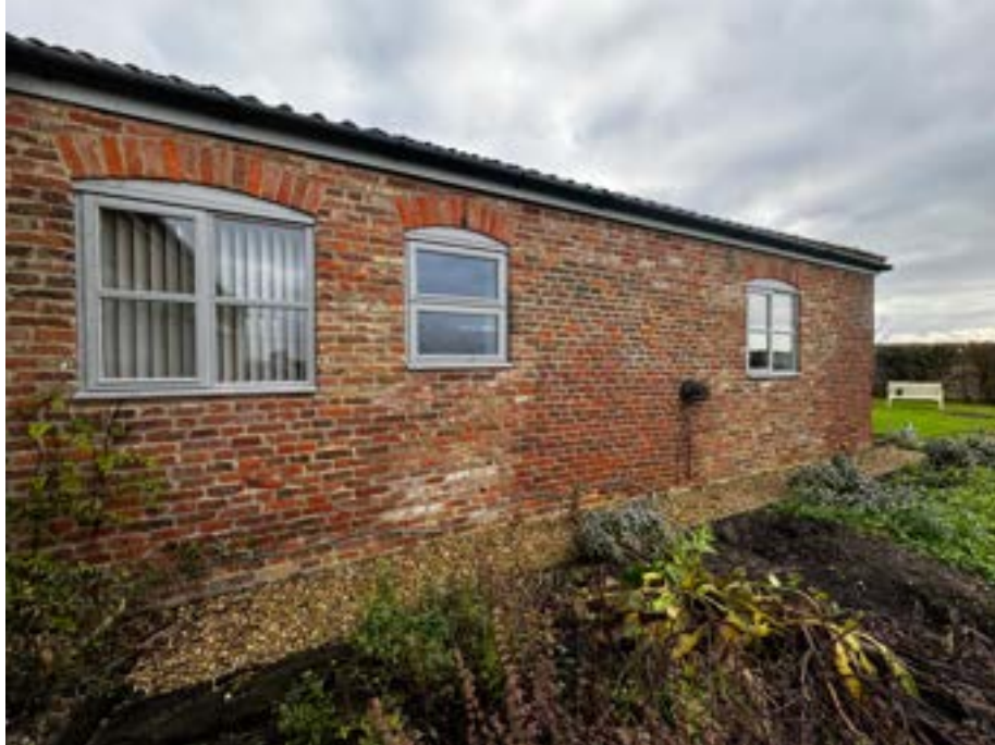
Image 3.0: External view of section previously converted.
