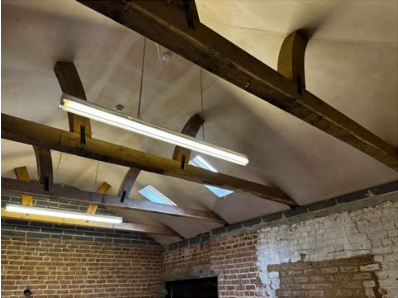
Image 8.0: View of ceiling to unconverted section of barn structure
