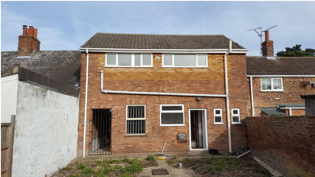
Rear Elevation – passageway on left hand side
