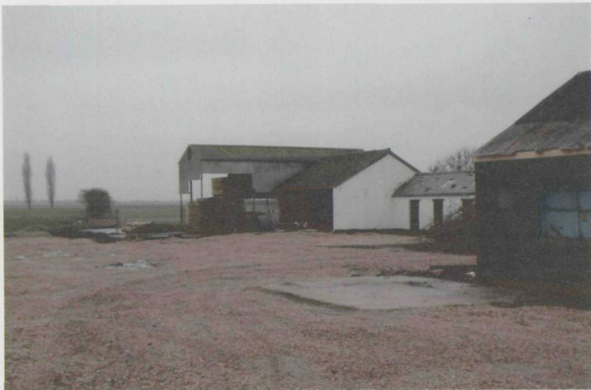
view south from centre of site
