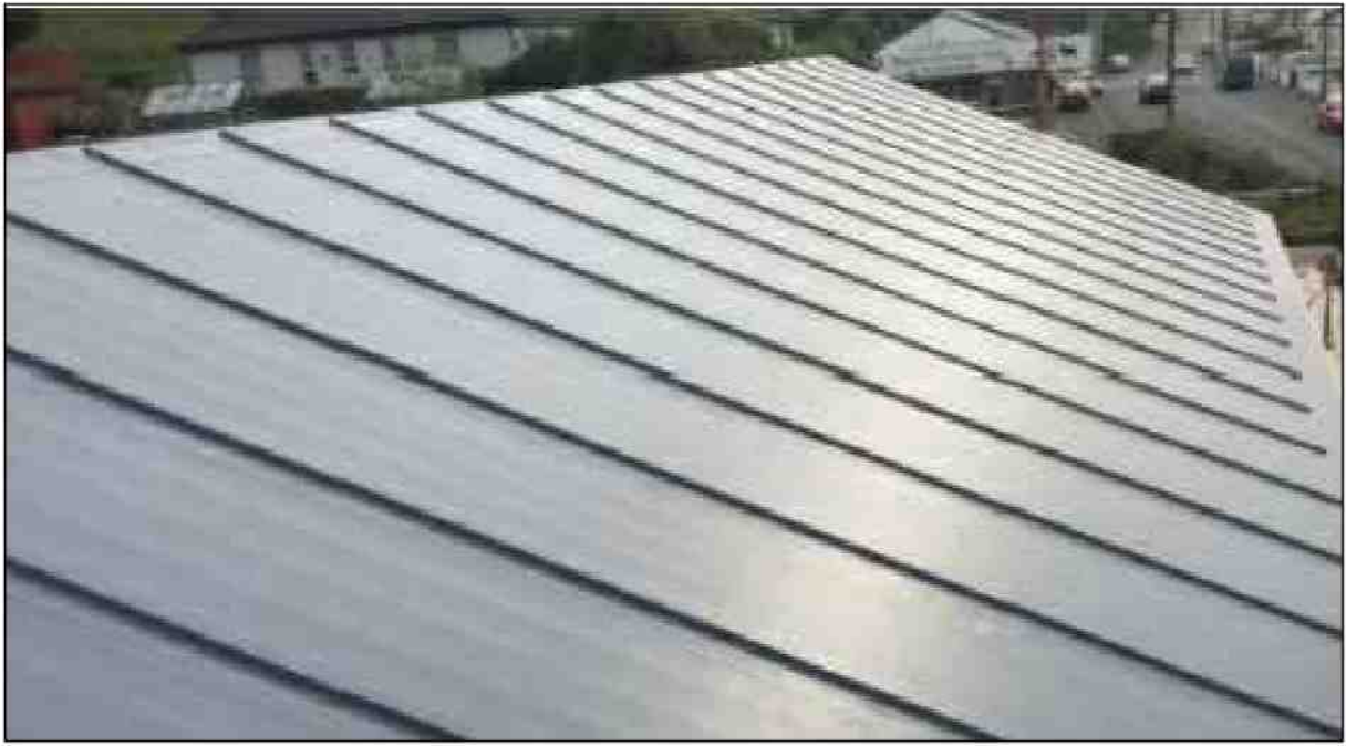
KINGSPAN INSULATED STANDING SEAM ROOFING N.T.S.
