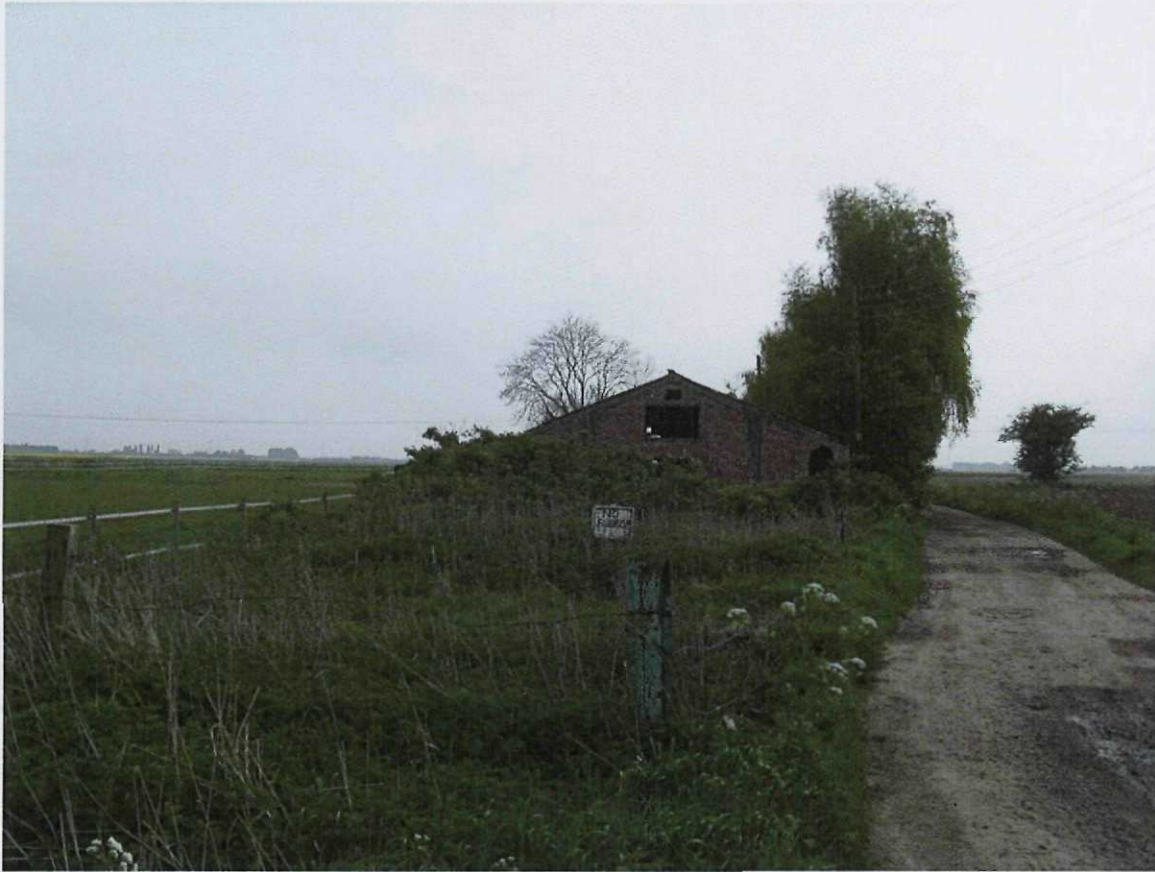
Existing Access Road and Side Elevation
