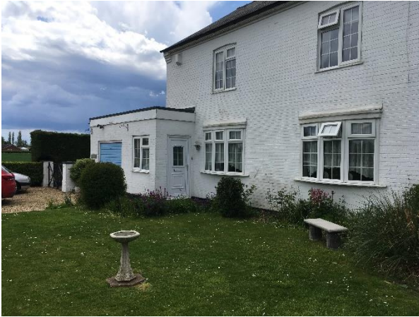
Fig 3. Front Elevation As Existing – painted white brick / white UPVC windows & doors
